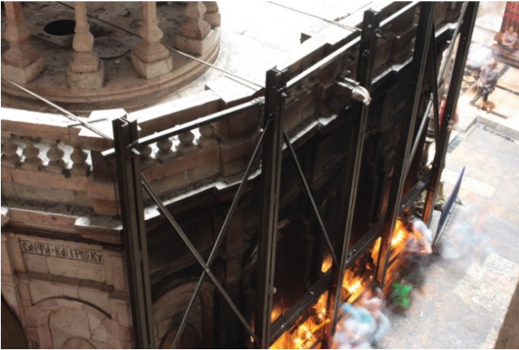
Fig. 15. The south façade of the Holy Aedicule in 2015 (© author)
