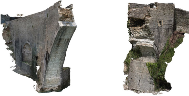
Fig. 13. 3D models of the remaining parts of the bridge (© author)
