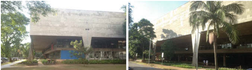
Fig. 3 Views of the concrete wall supported by the trapezoids shaped columns. Source Images from the authors
