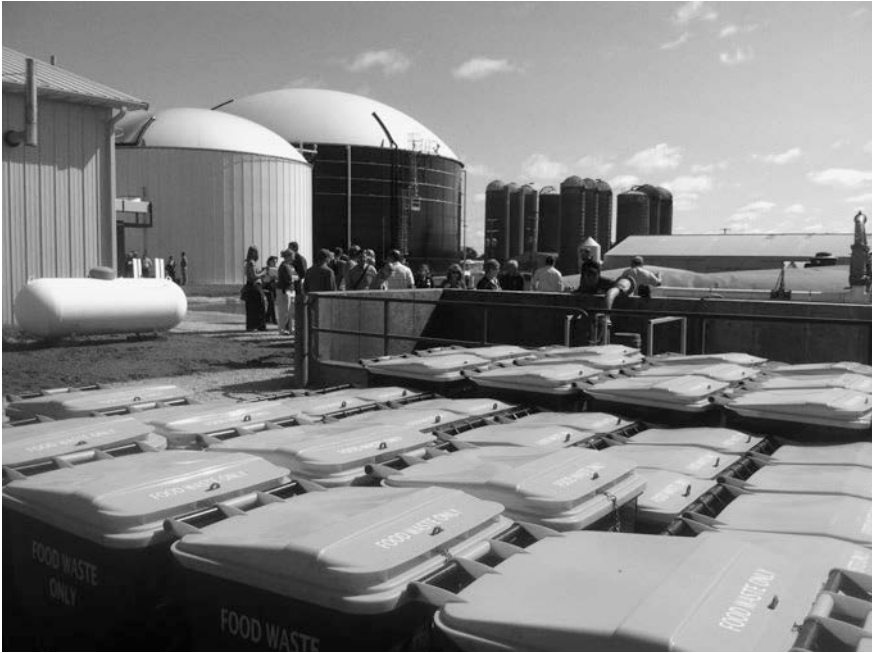
Fig. 1 MSU south campus anaerobic digester. The large tanks in the background are the digester and digestate storage tanks; the lidded containers in the foreground are used for feedstock delivery
