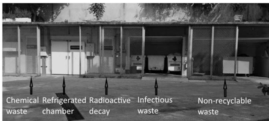
Fig. 1 Installation for storage wastes before final destination at Medicine Building Complex. The chemical storage room is not shown (Faculty of Medicine—USP 2017)
