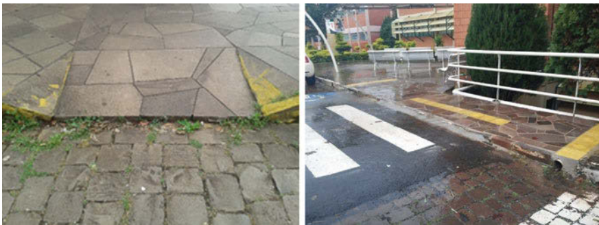
Fig. 2 Ramp before and after modifications
