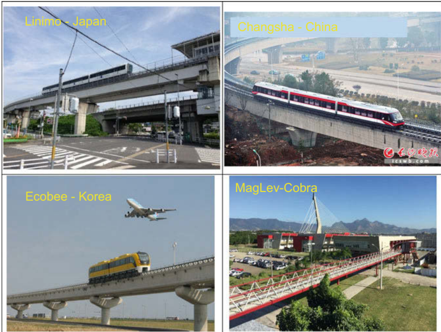
Fig. 4 Comparison of the elevated lines of the EML urban MagLev projects in commercial use and the MagLev-Cobra (SML) elevated line: slimmer structure
