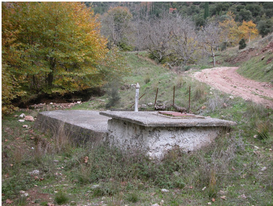
Fig. 3 Intake of water from a spring in a remote mountainous area in Greece
