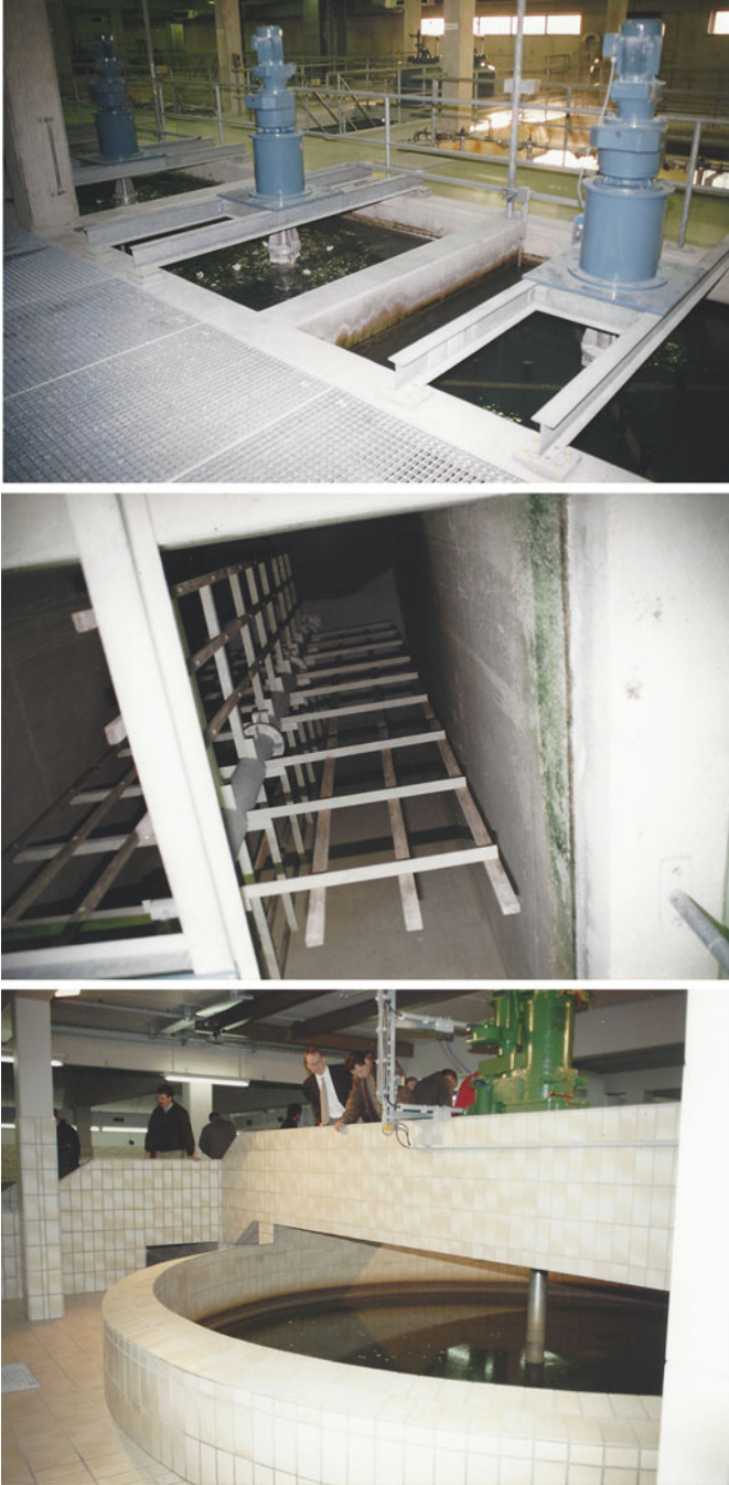
Fig. 7 Top , Tapered flocculation tanks; Centre , mixing device in flocculation tank; Bottom , flocculation tank in Wuppertal (Germany)
