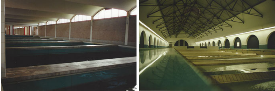
Fig. 10 Rapid sand filtration in the Netherlands ( left ) and in Germany ( right )
