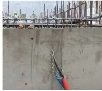
(b) residual sensor cables after concrete pouring and hardening
