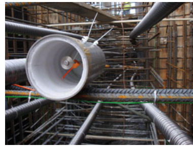
(c) detail of "no-stress" strain enclosure
