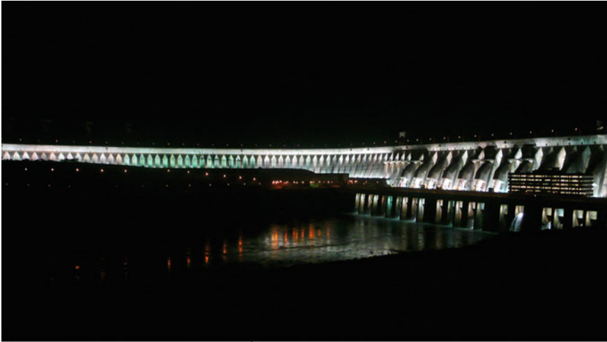
(a) General view of the concrete dam
