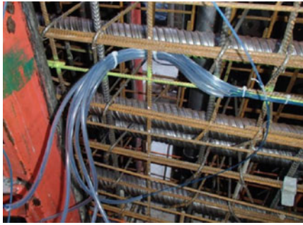
(a) fibre optic cable sensors secured in place and grouped together
