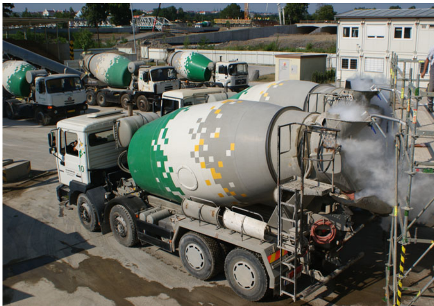
Fig. 6.1 Photograph of typical in-site application of LN cooling in concrete truck (courtesy of O. Kunc, TBG Metrostav)
