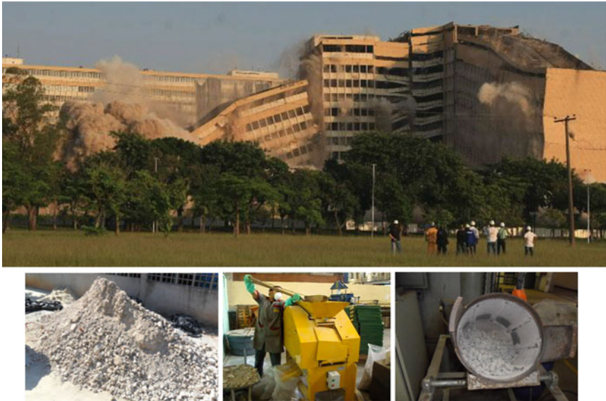
Fig. 10.3 (Up) Demolition of hospital section, Ilha do Fundão, Rio de Janeiro, Brazil; (down left to right) homogenization process, grinding process with a crusher and autogenous cleaning
