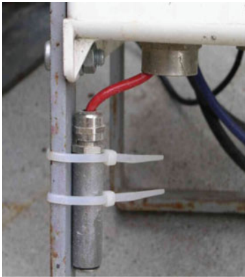
(i) placement close to the concrete surface with shielded sensor
