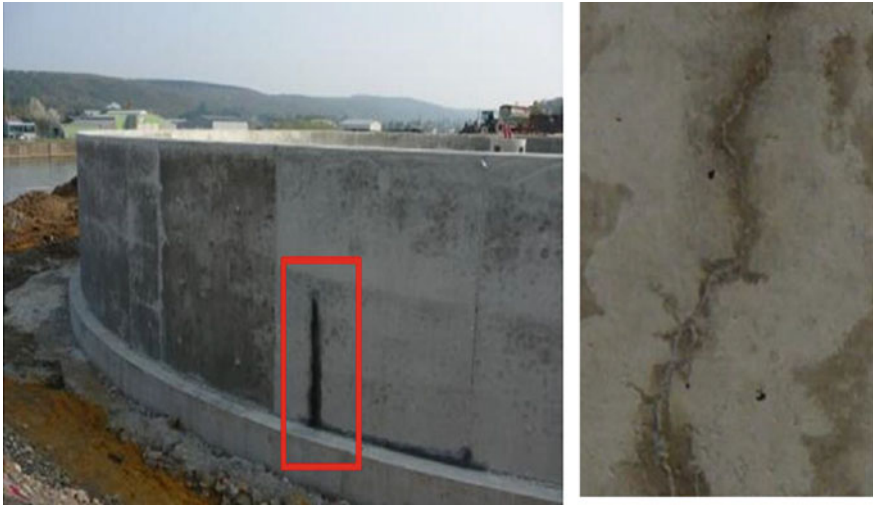
Fig. 8.4 Water treatment plant showing cracking due to the restrained shrinkage at early age and some self-healed cracks (photograph: A. Darquennes)
