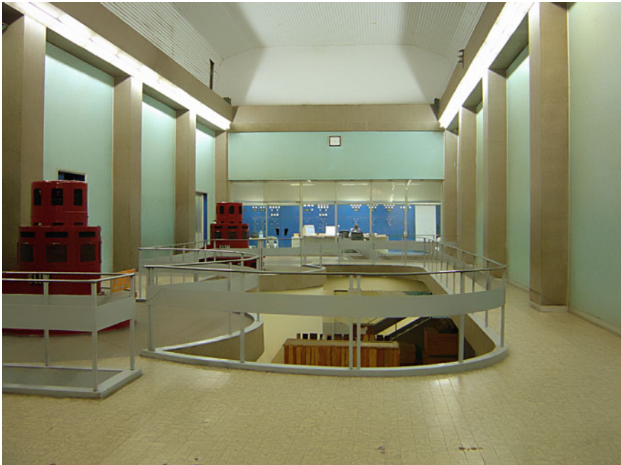
Fig. 2.3 Rehabilitated control room relates to the Abd El Al power plant
