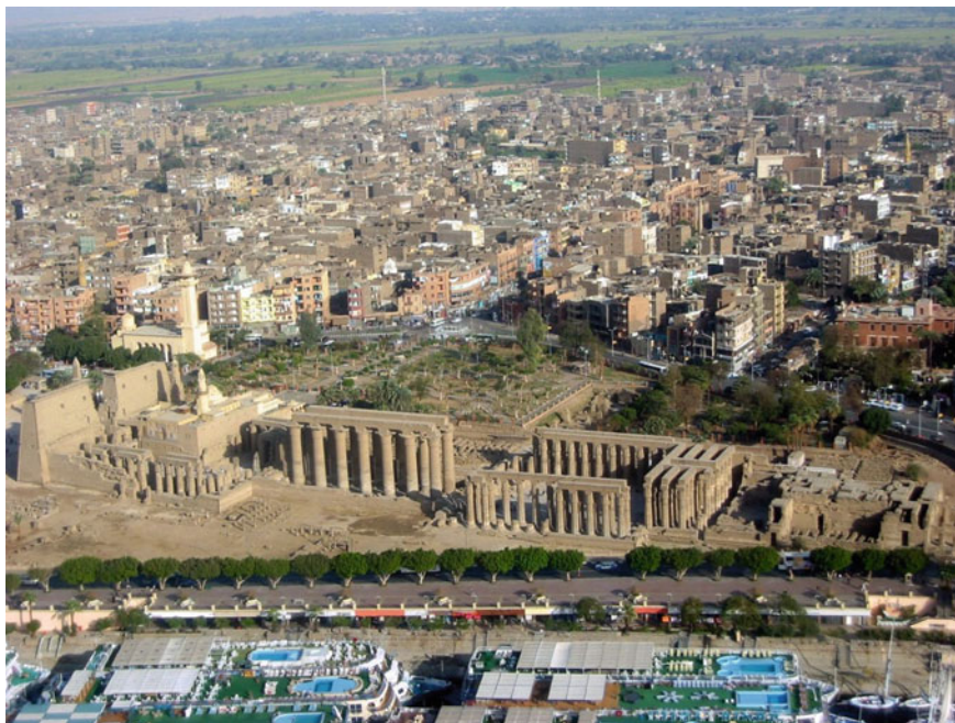
Fig. 11.3 An aerial view on Luxor Temple where cruise boats and the corniche are at the bottom while the compatibility with the surrounding buildings is shown at the top of the image (the authors)
