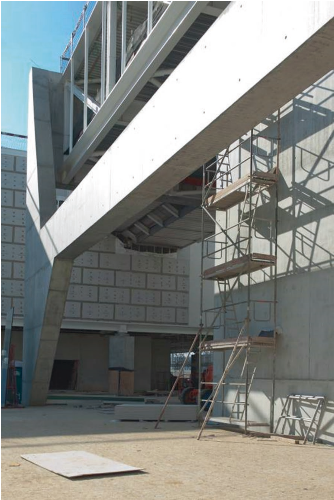
Fig. 52 Auditorium under construction before the finishing phase
