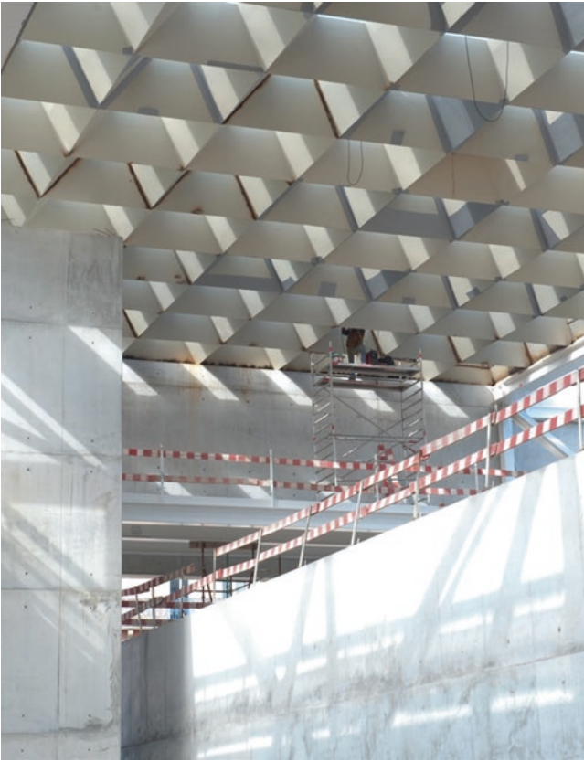
Fig. 17 Skylights of the auditorium under construction
