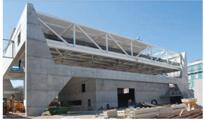
Fig. 18 Auditorium under structural construction phase
