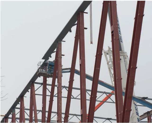
Fig. 14 Wall structure under construction
