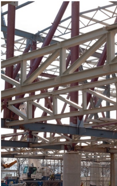
Fig. 4 Main structure of the museum during the construction from the outside
