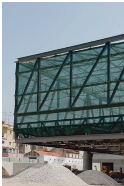
Fig. 39 Main building's external wall under construction
