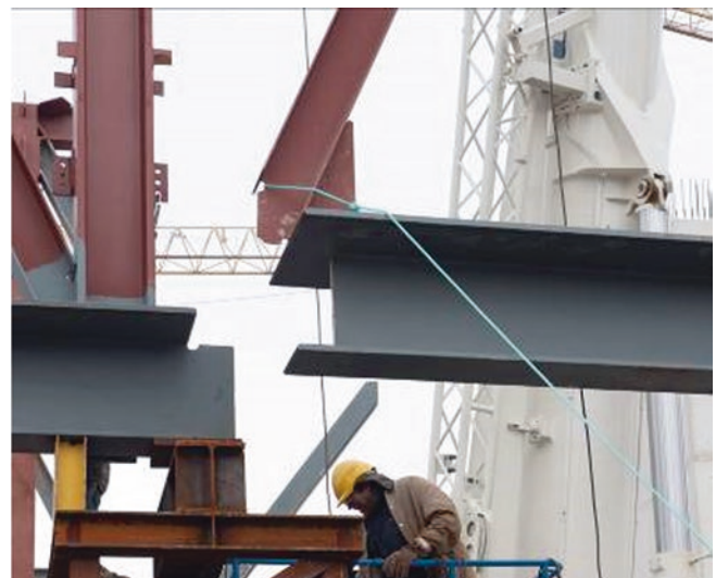
Fig. 30 Detail of the beam of the main building's external wall under construction
