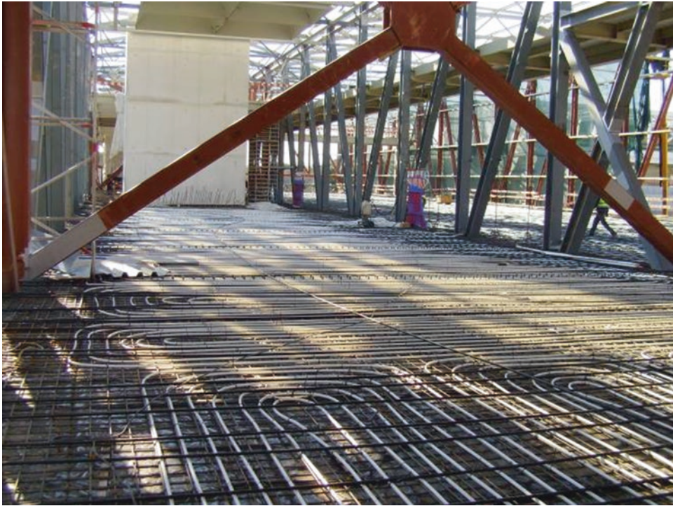
Fig. 88 Floor heating system
