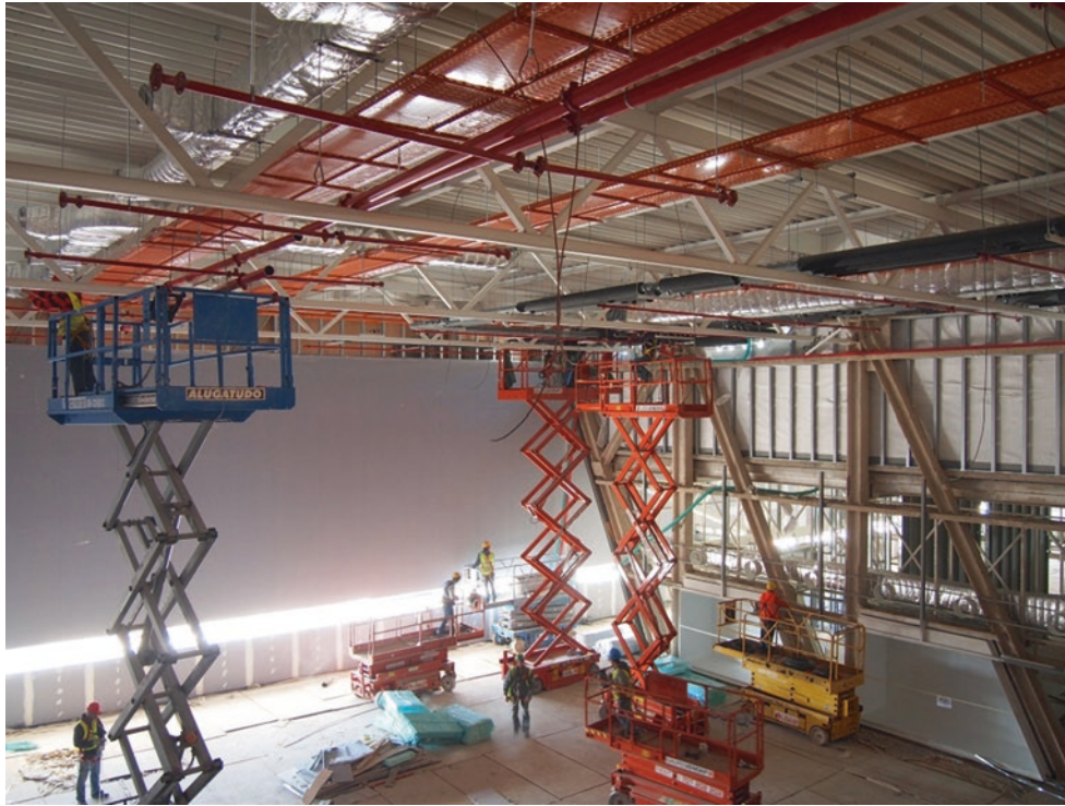
Fig. 5 Physical space for the service installations. (Photo by Raimundo Constância)
