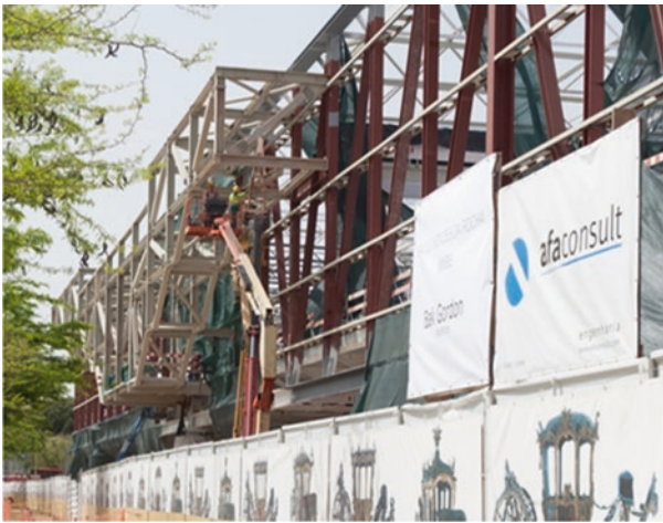
Fig. 37 Main wall building under construction
