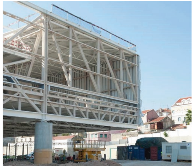
Fig. 15 View from the exterior in the structural construction phase
