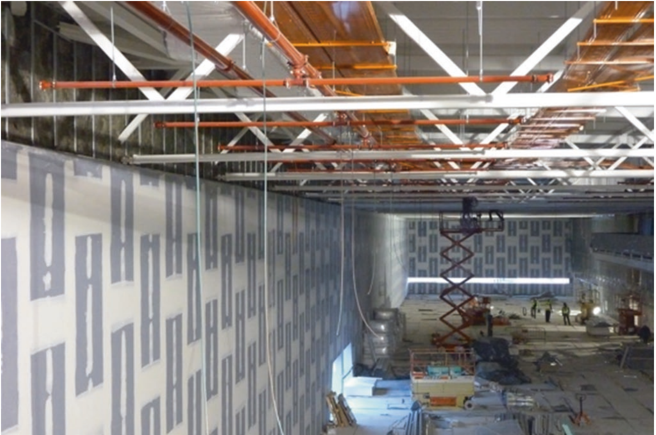
Fig. 77 Infrastructures construction phase
