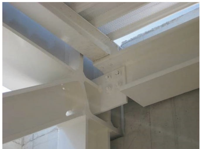
Fig. 48 Detail of the connection of the steel structure with the concrete wall - cross section
