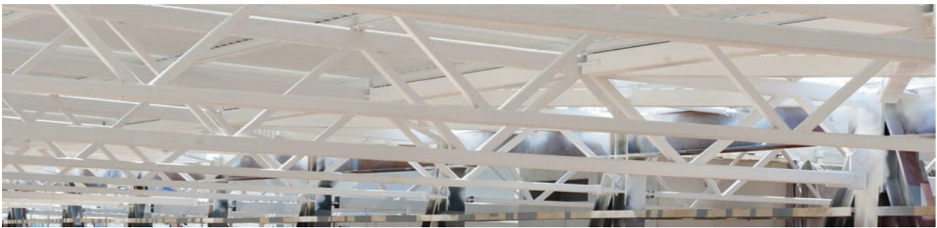
Fig. 11 Roof structure under construction
