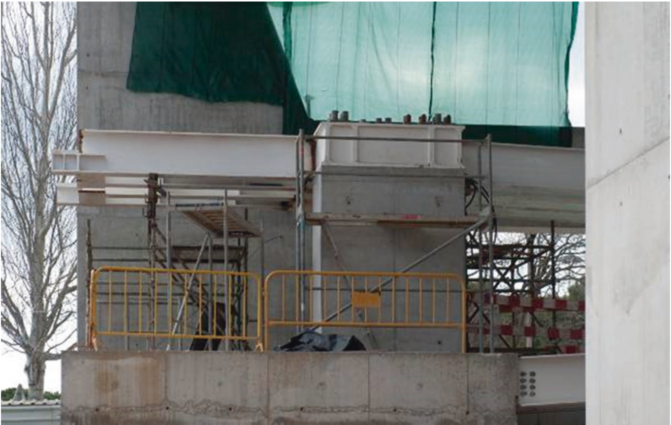
Fig. 69 Walkway under construction
