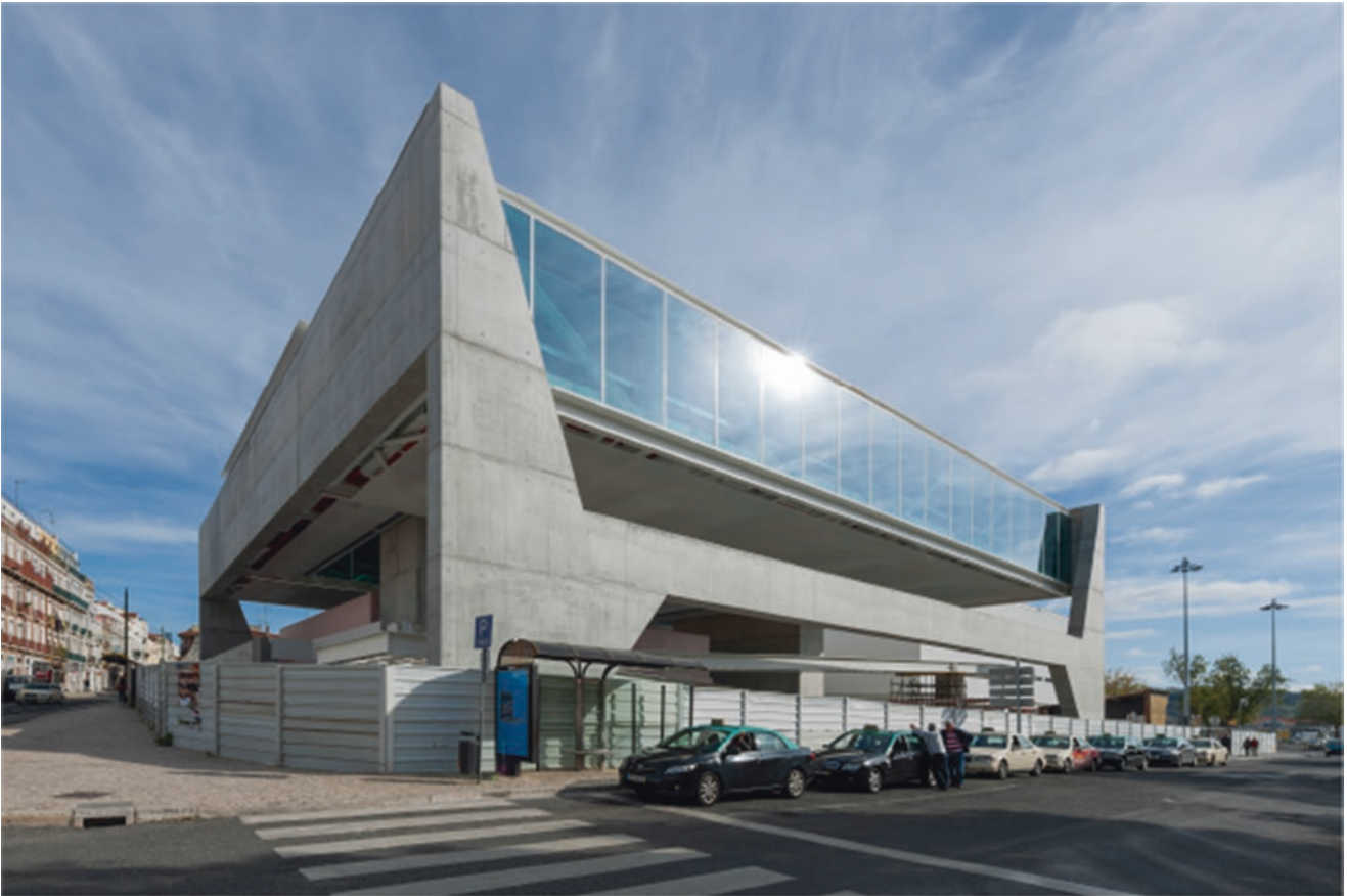
Coach Museum Auditorium External view from Junqueira street Copyright Arménio Teixeira
