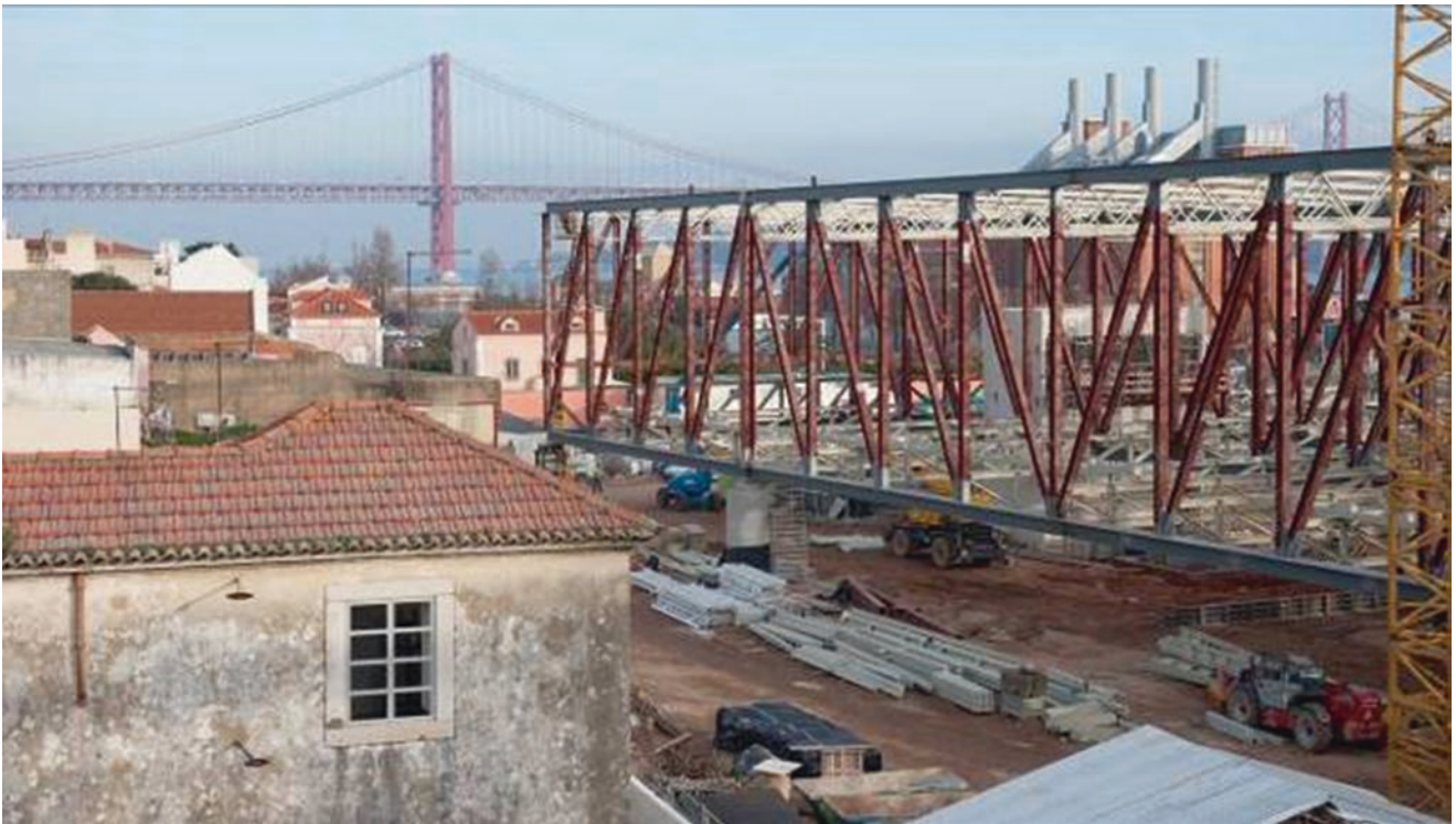
Fig. 24 View of the main building under structural construction phase from the second level of the auditorium
