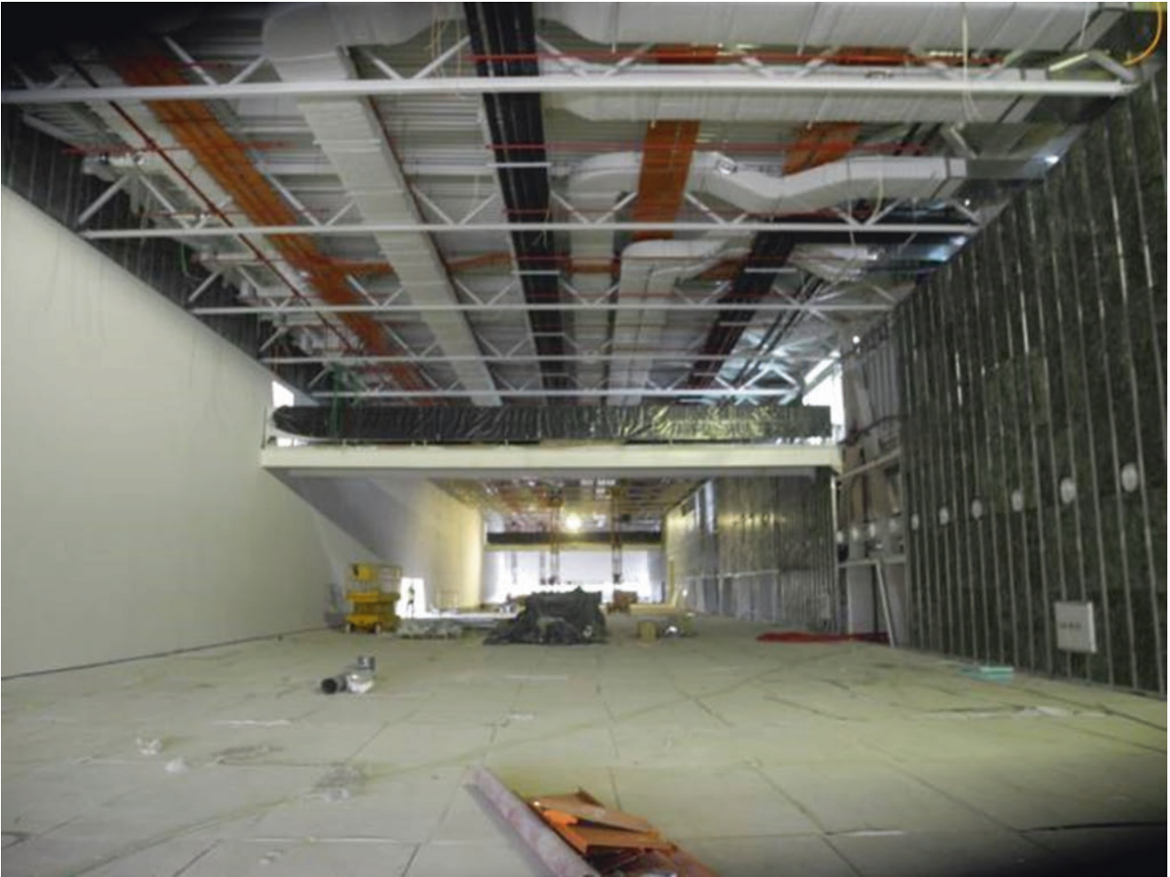
Fig. 85 Main room in the finishings construction phase
