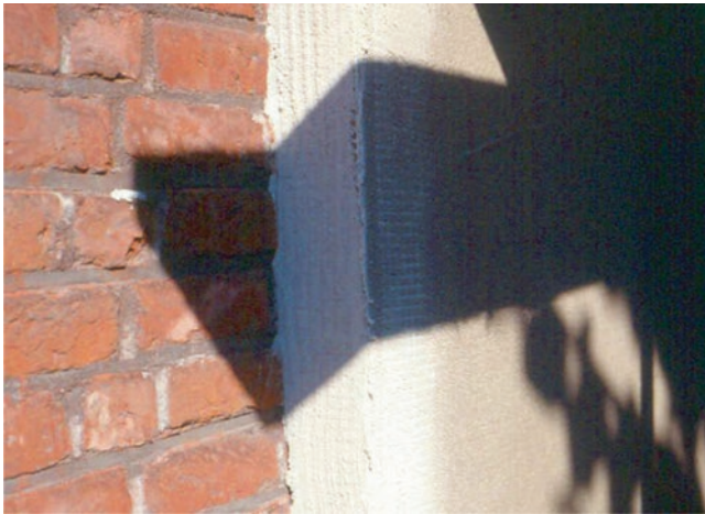
Fig. 3 EIFS outside insulation
