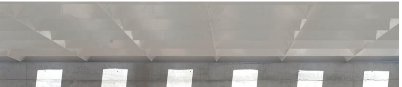
Fig. 20 Skylights of the auditorium under construction
