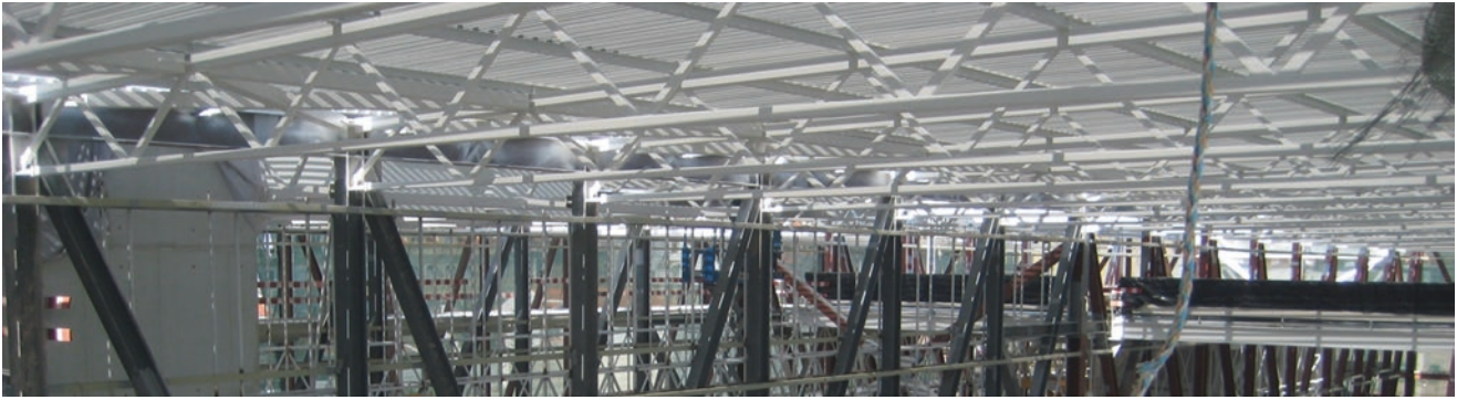
Fig. 28 Roof structure under construction
