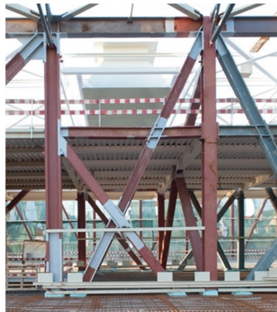
Fig. 40 Main building's external wall module under construction
