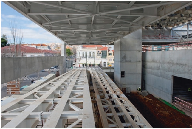
Fig. 8 Ramp under construction
