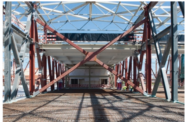
Fig. 38 Main wall interior under construction before the concreting phase
