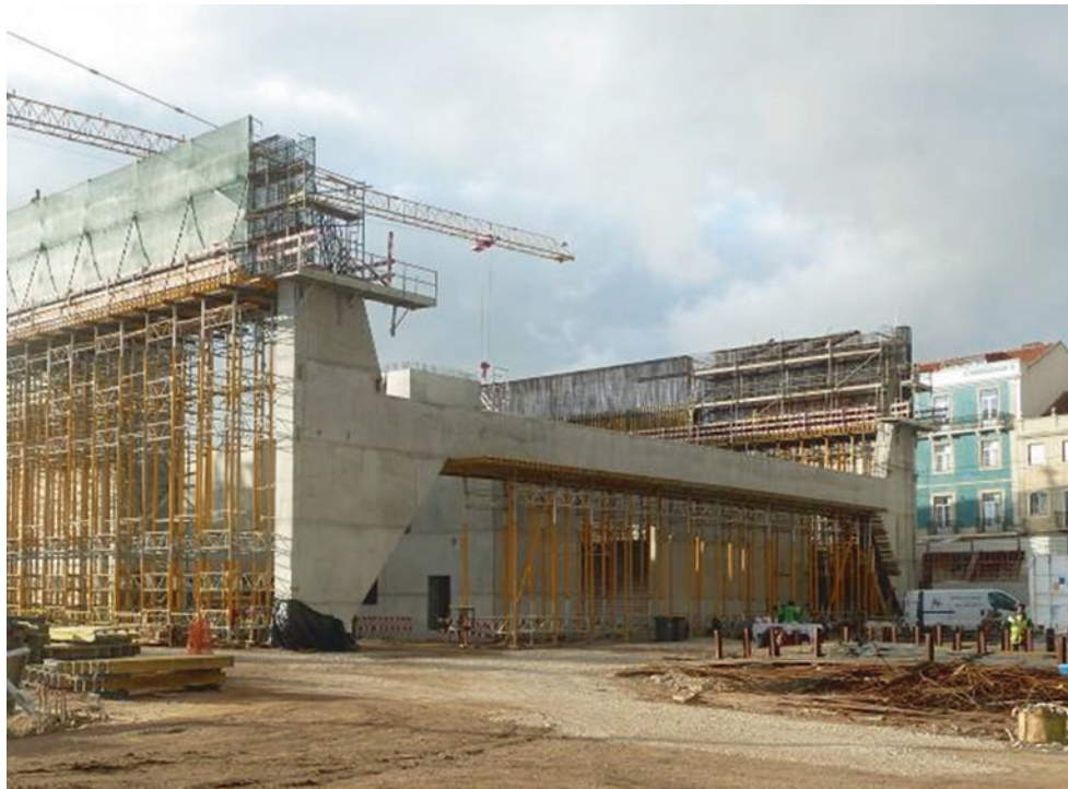
Fig. 43 Auditorium structure under construction
