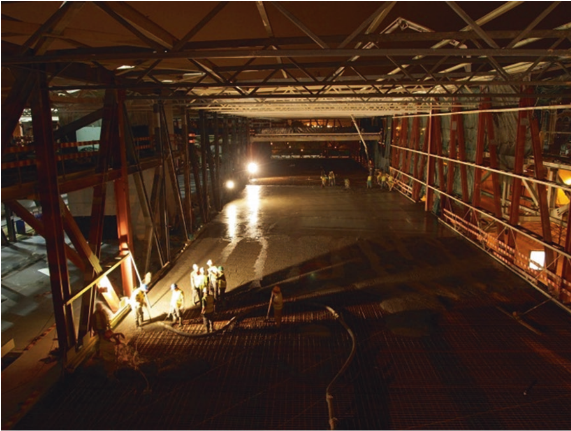
Fig. 2 25 m × 100 m slab finished directly. (Photo by Raimundo Constâncio)
