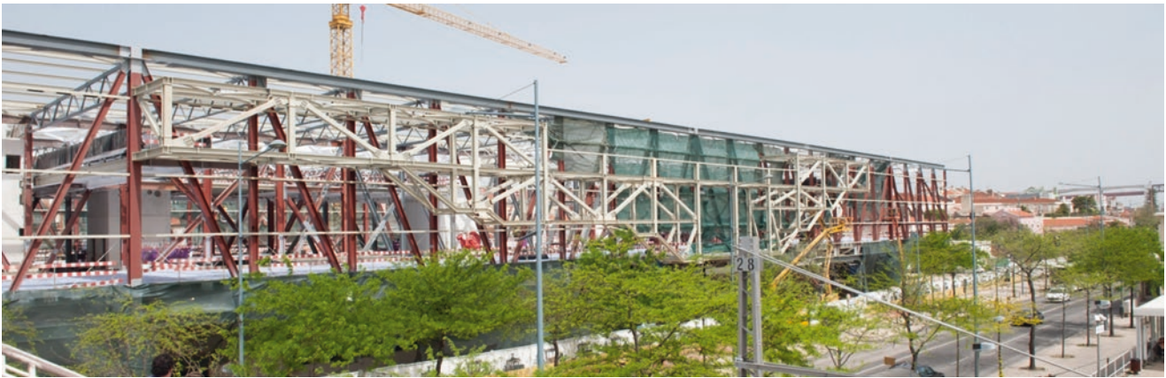
Fig. 23 Street view of the main building under structural construction phase
