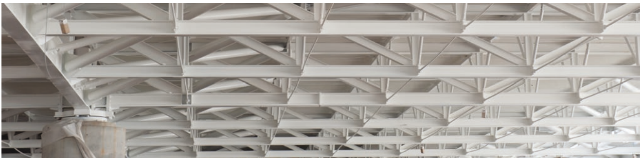
Fig. 35 View of the main building slab from the lower level
