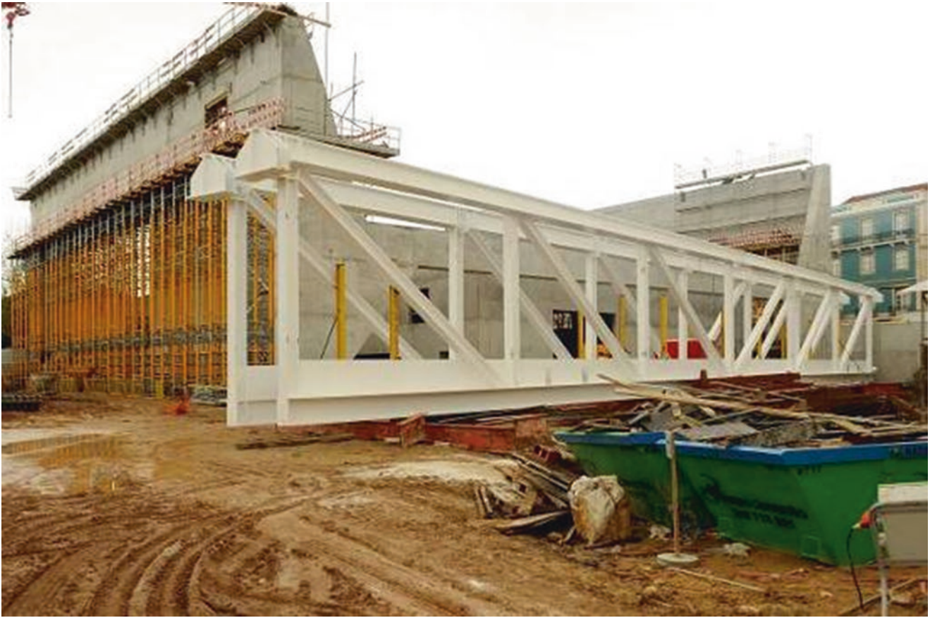
Fig. 50 Auditorium truss structure before placement
