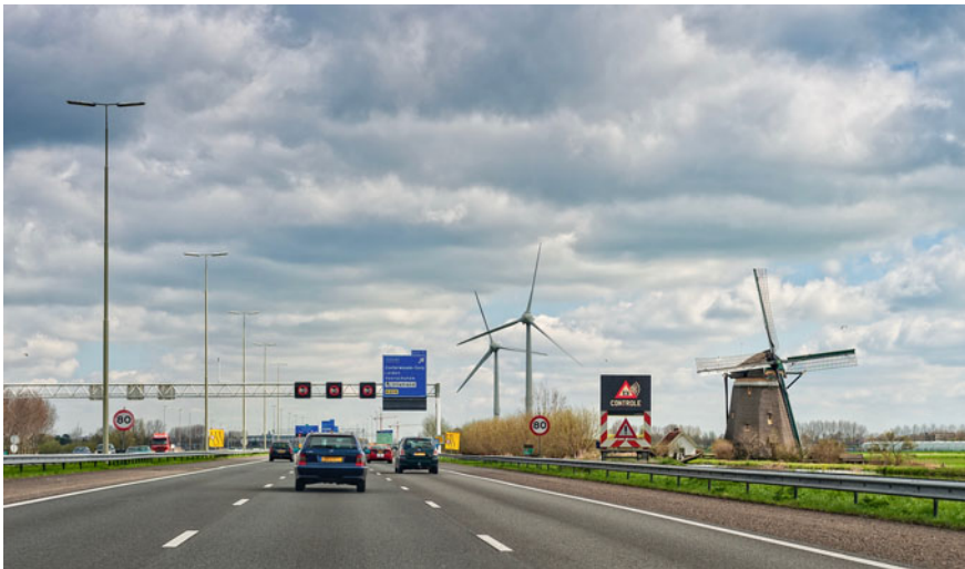
Fig. 10.1 A road stretch in A4 freeway, close to Leiden, the Netherlands (courtesy of Rijkswaterstaat, Photo: Essencia Communication/Rob de Voogd)
