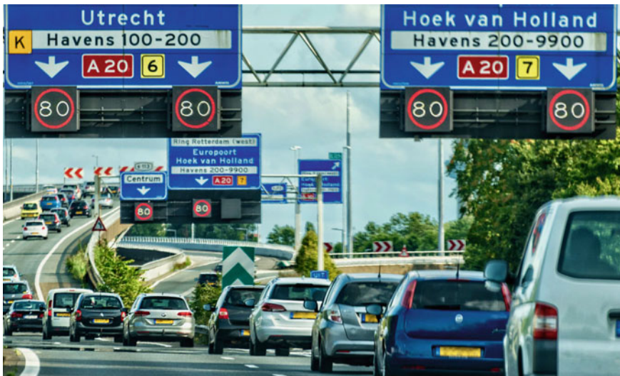
Fig. 1.10 Variable speed limits at the junction Kleinpolderplein of the A13 and A20 freeways, the Netherlands (courtesy of Rijkswaterstaat, Photo: Essencia Communication/Rob de Voogd)
