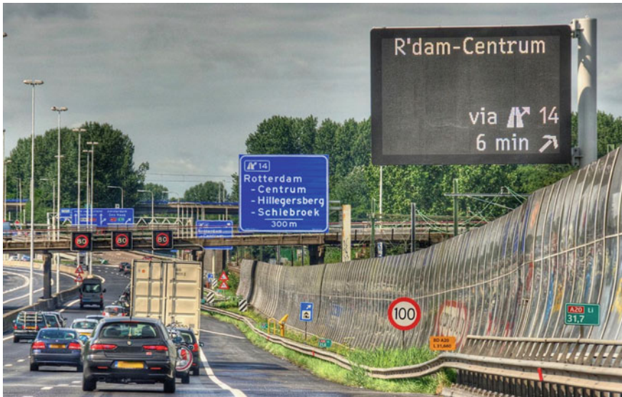
Fig. 1.11 Routing indications in A20 freeway, close to Rotterdam, the Netherlands (courtesy of Rijkswaterstaat, Photo: Essencia Communication/Rob de Voogd)
