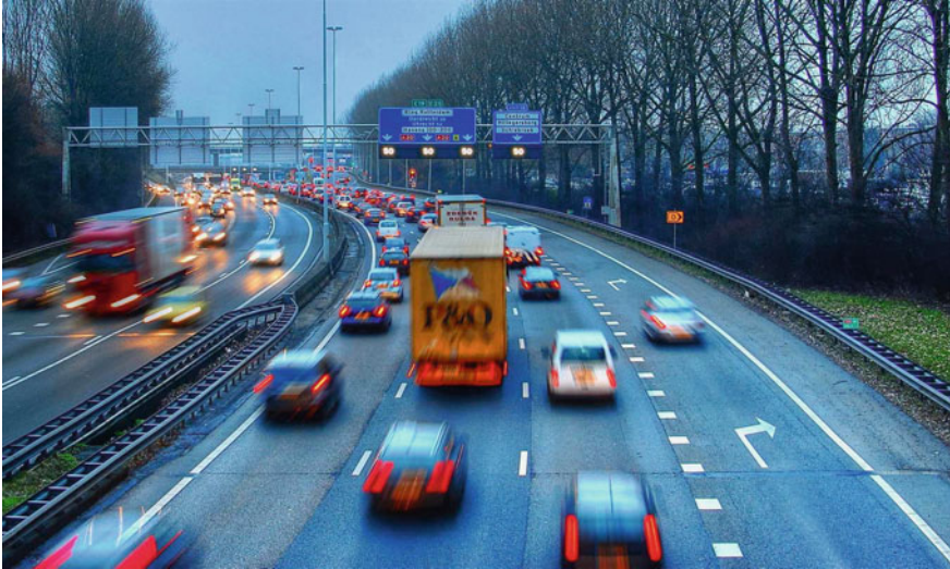
Fig. 8.4 Variable speed limits in A20 freeway, close to Rotterdam, the Netherlands (courtesy of Rijkswaterstaat, Photo: Essencia Communication/Rob de Voogd)
