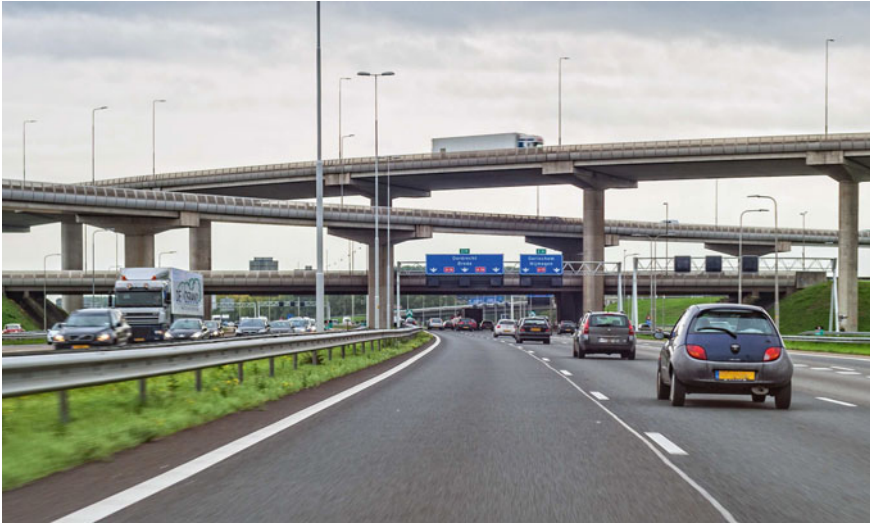
Fig. 9.1 Junction Ridderster of the A15 and A16 freeways, the Netherlands (courtesy of Rijkswaterstaat, Photo: Essencia Communication/Rob de Voogd)
