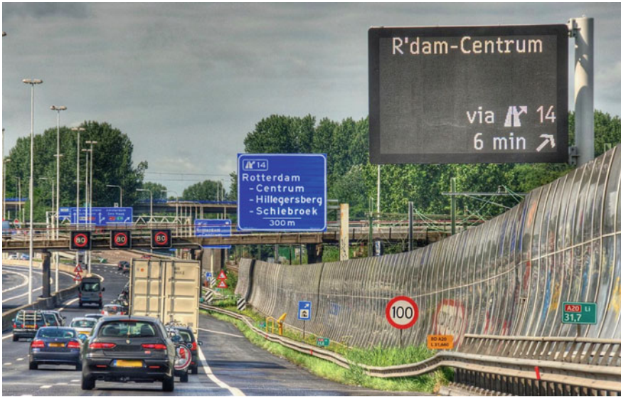
Fig. 1.11 Routing indications in A20 freeway, close to Rotterdam, the Netherlands (courtesy of Rijkswaterstaat, Photo: Essencia Communication/Rob de Voogd)
