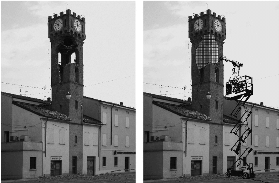
Fig. 8. Simulation of an on-site rapid prototyping intervention of the Novi of Modena's clock tower, in the situation after the first earthquake shock of 2012. It collapsed as a result of a subsequent shock (photo by prof. Pietromaria Davoli and elaboration by Sara Codarin).
