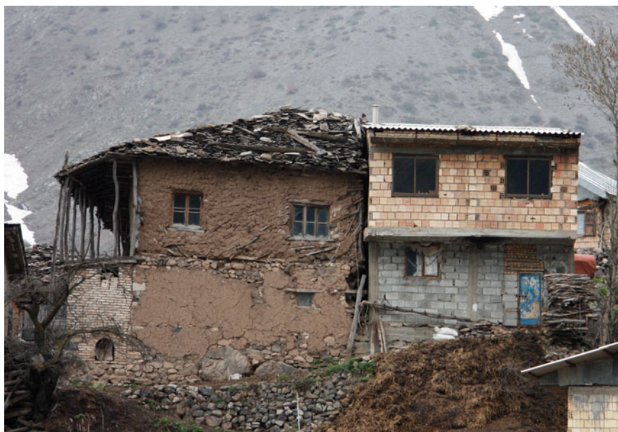
Fig. 8.2 Contrast between the traditional and RHSP constructed houses, (A traditional house of Nater being cut in half for a RHSP house to be constructed), author, March 2017
