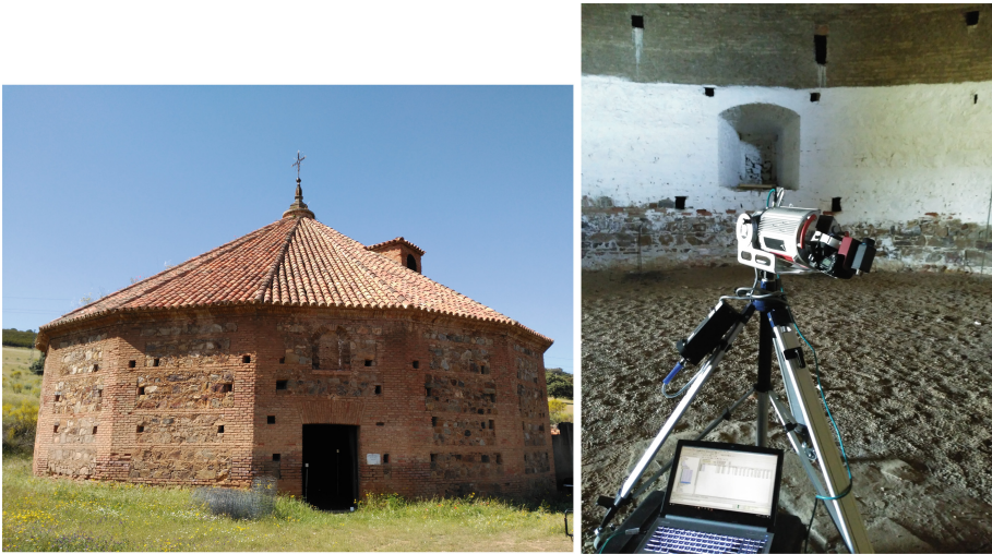
Fig. 4. Baritel de San Carlos: exterior and interior views.
