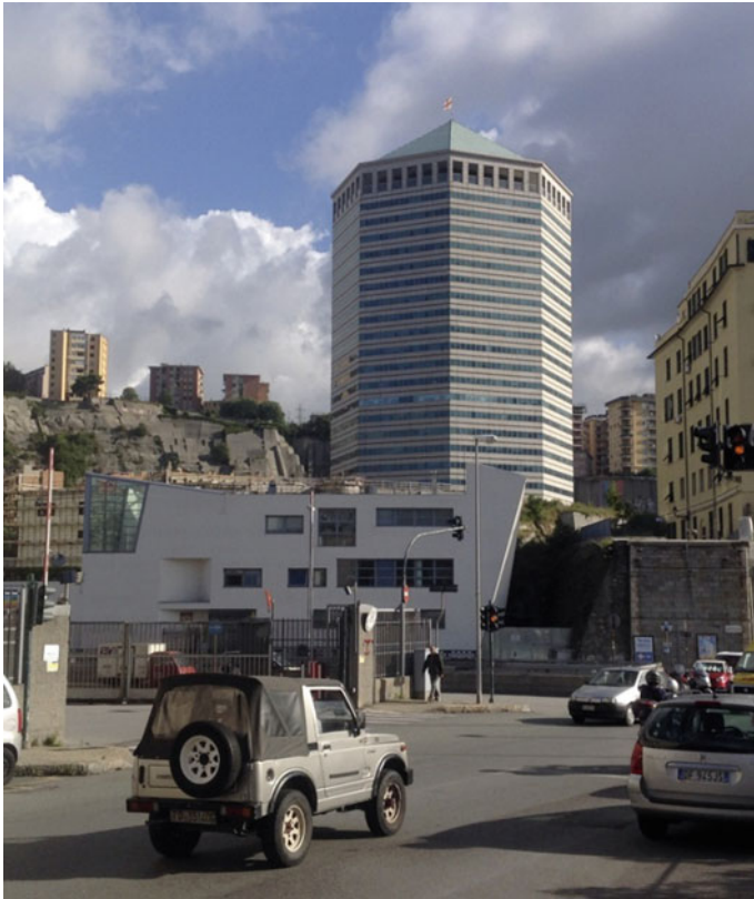
Fig. 1 The skyscraper called “Il Matitone”. The Association Genova Smart City has promoted a study to optimize energy consumption in this building. Photo G. Sergi 2016
