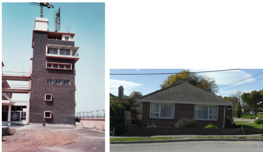
Fig. 16.10 Settlement and rotation of a tall structure and a residential structure due to soil liquefaction
