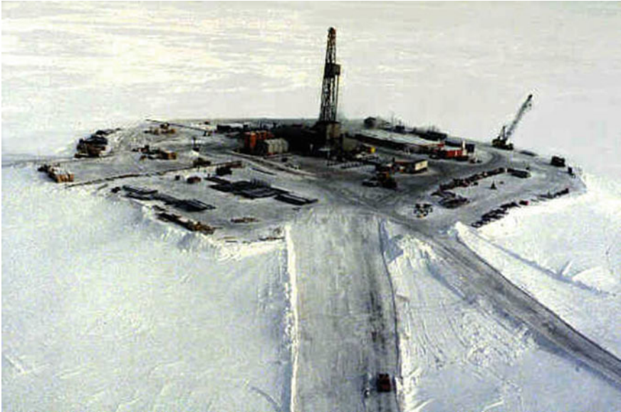
Fig. 6.3 Mars Ice Island, Beaufort Sea Alaska. Image shows a 60-day exploratory well built 8 km (5 mi) offshore of Cape Halkut near the National Petroleum Reserve in Alaska (NPRA), an area of land on the Alaska North Slope owned by the United States federal government and managed by the Department of the Interior, Bureau of Land Management (BLM). (Photo courtesy of Bureau of Ocean Energy Management)
