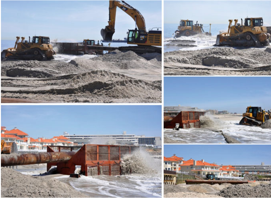
Fig. 15.6 Following hurricane sandy, the U.S. Army Corps of Engineers replaced roughly 6.1 million \text{m}^3 (8 million \text{yards}^3 ) of sand to repair and restore engineered beaches along the Atlantic coast of Monmouth County, NJ (courtesy of U.S. Army Corps of Engineers)
