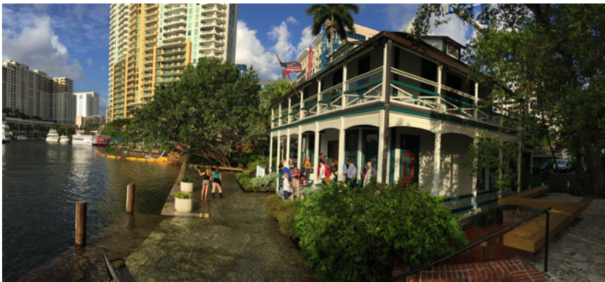
Fig. 14.1 “Nuisance flooding” of the historic Stranahan House, Ft. Lauderdale, October 2015 (Photo-C. R. Nichols)
