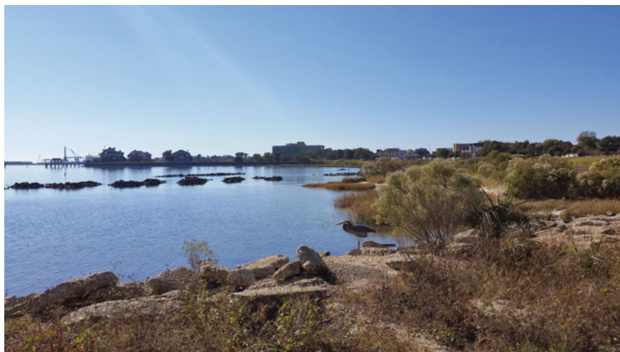
Fig. 11.7 View of project greenshores showing breakwaters. Credit Darryl Boudreau, The Nature Conservancy
