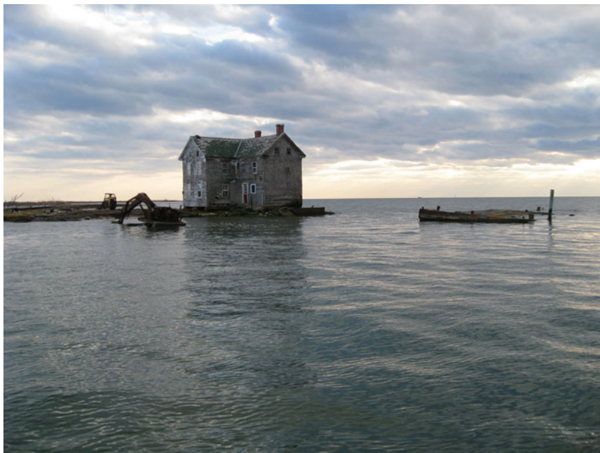
Fig. 15.5 The last house on Holland Island, which was built in 1888, collapsed into the Bay in October, 2010. This photograph of the Holland Island, which is barely discernible today, was taken on November 9, 2008 (courtesy of the Chesapeake Bay Foundation, Photo by Chuck Foster)
