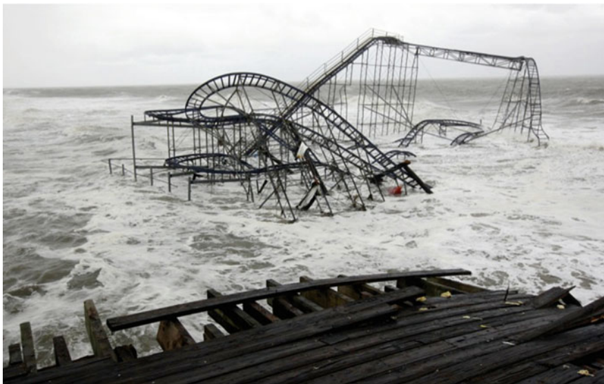
Fig. 5.7 Inundated boardwalk amusement park in Atlantic City, New Jersey in the aftermath of Hurricane Sandy (Photo of roller coaster on Casino Pier in Seaside Heights, NJ courtesy of Star Ledger)
