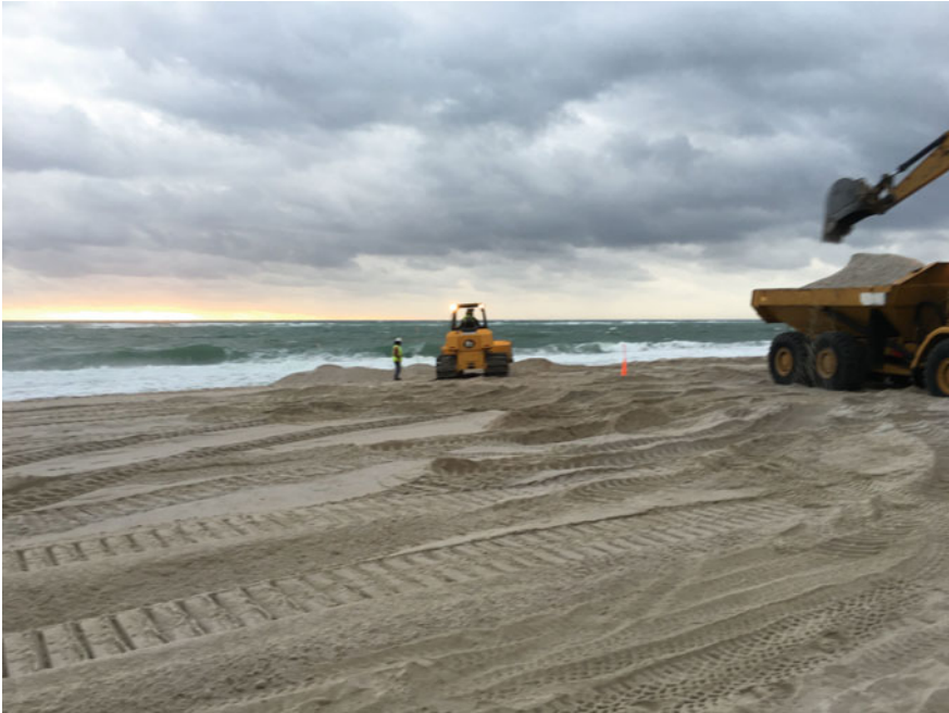
Fig. 5.8 Large-scale beach re-nourishment project, Pompano Beach, Florida January 2016. The project took 3-months to complete (Courtesy of L. D. Wright)
