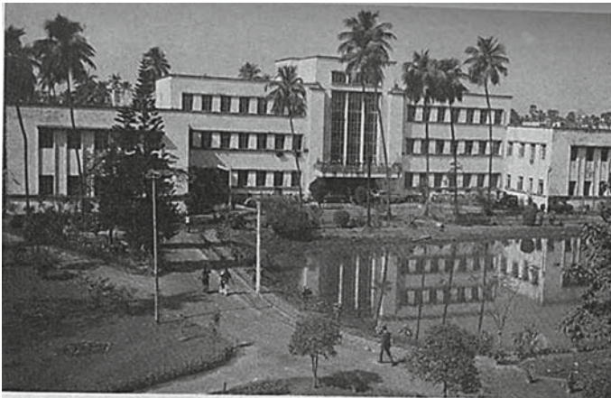
Fig. 1.3 The Indian Association for the Cultivation of Science (IACS) in Calcutta (Raja S.C. Mullick Road), the institution where C.V. Raman discovered the effect named after him. Note that the original building in which the discovery actually took place was then located on Bow Bazar Street, also in Calcutta. It seems that no picture exists of the IACS building at that time [3]
