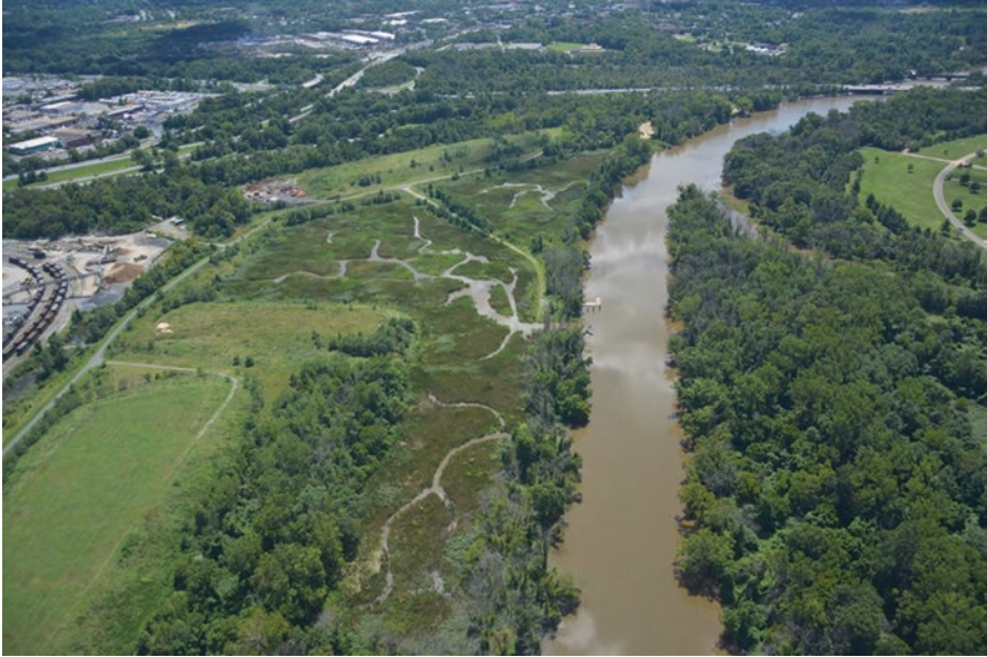
Fig. 9.2 The Bladensburg Wetlands was a landfill known as “ANA 11” until the Maryland State Highway Wetland Mitigation Project transformed the area into this natural water filter and wildlife habitat in 2008 (Photo courtesy of the Anacostia Watershed Society, used by permission)
