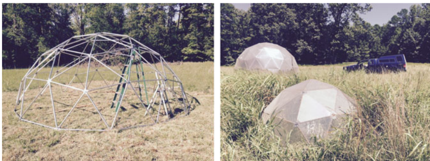
Fig. 3.19 (Left) The frame for the 6 m dome. (Right) The completed 6 m dome is at right. The 2.4 m dome is seen in front
