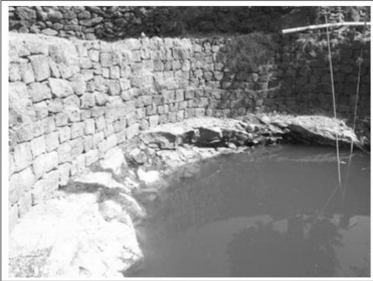
Fig. 9.2 A spring converted to a spring-cum-well in the Western Ghats. The spring outlet is on the left behind the stone wall, and can be seen emerging into the well. This type of conversion from a groundwater to surface water source can lead to contamination of the water. The colour of the water is green which indicates algal growth. It is recommended that a springbox be built at the outlet so that groundwater can be harvested prior to any potential surface contamination, with the overflow collected in the open well for other uses. Also, as this is a contact spring type, there is no increase in water yield due to excavation of the well
