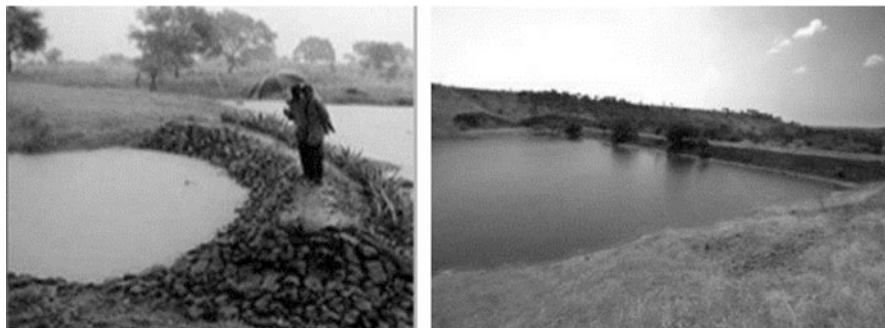
Fig. 18.9 Direct surface recharge through percolation tanks in Satpura Mountainfront area in Maharashtra
