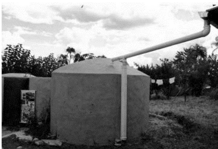
Fig. 18.6 A rainwater collection tank made of ferro-cement. Source: Dolman and Lundquist (2008)
