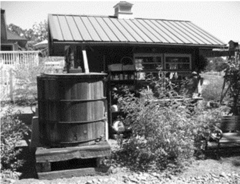
Fig. 18.2 Roof-top rainwater harvesting in rural areas
