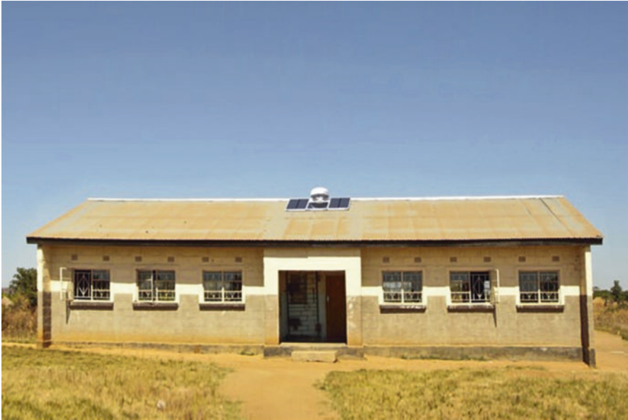
Fig. 5.3 A ground-station for OneWeb satellites pictured on the roof of a rural school. (Image courtesy of OneWeb)
