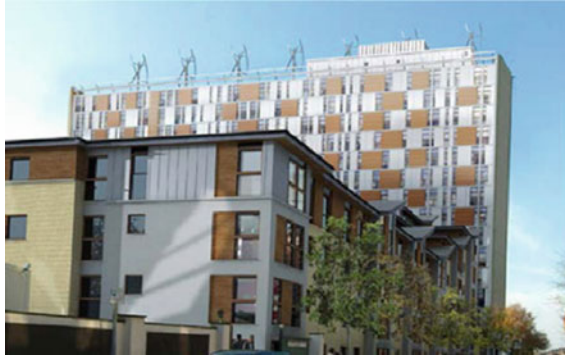
Fig. 6 Placement on flat roof of a residential building in accordance with the character of the building [23]
