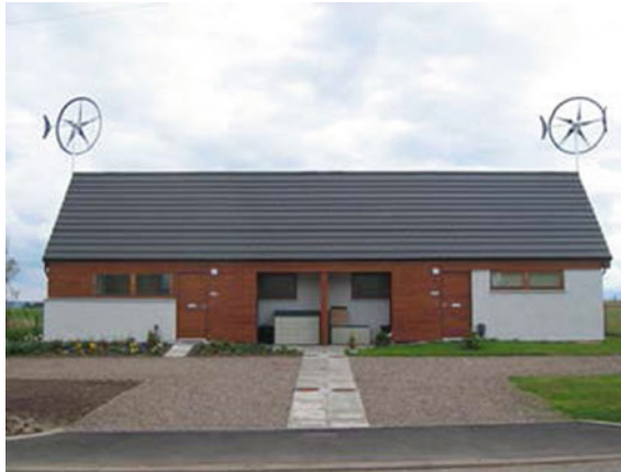
Fig. 7 Positioning of turbines with respect to the symmetry character of the building [19]
