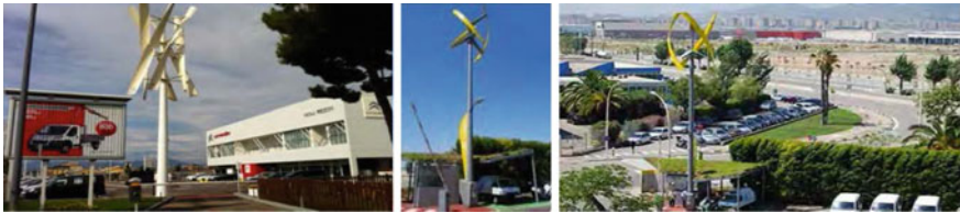
Fig. 3 Sensitive siting: micro wind siting seems more appropriate on buildings and structures that already have a technological character or at their open spaces such as parking areas at commercial or industrial centres [23]
