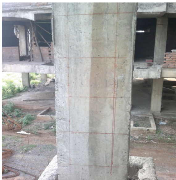
Fig. 5 Gridlines marked on the surface of column
