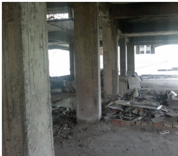
Fig. 4 Internal view of the old building to be tested
