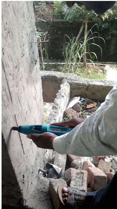
Fig. 9 Silver schmidt digital rebound hammer used on the column
