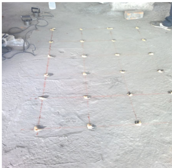
Fig. 6 Slab surface prepared for the ultrasonic test
