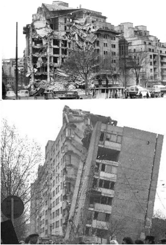
Fig. 1 Partial collapse of some buildings in Bucharest after the 1977 earthquake (photo by Ene 1977)
