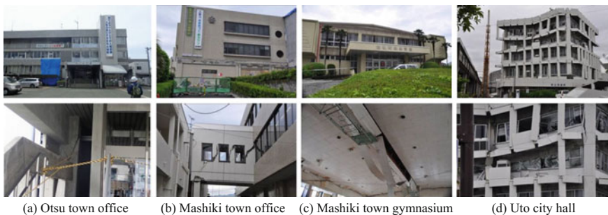
Fig. 1 Damage of disaster management facilities due to the 2016 Kumamoto earthquake
