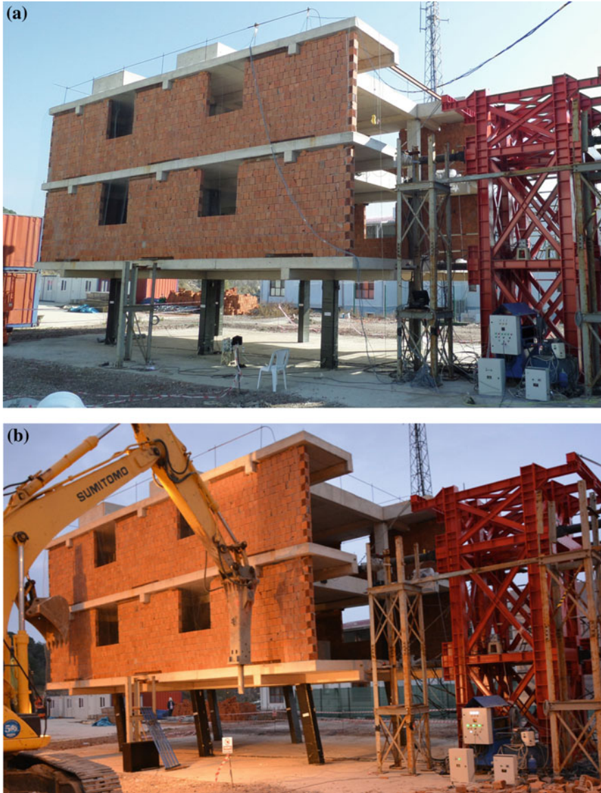
Fig. 3 General views of the retrofitted building a before and b after the test
