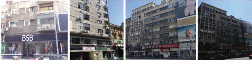
Fig. 6 Buildings with different function ground floors relative to the upper levels
