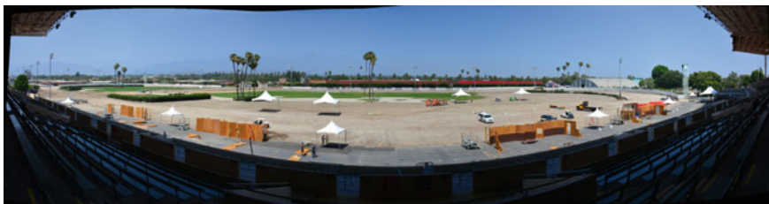
Fig. 12 Course construction progress 9 days before the event
