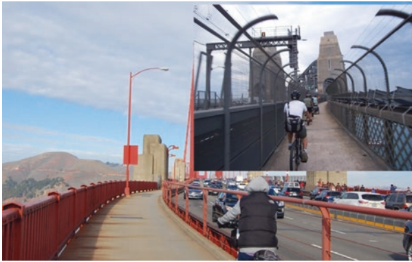
Fig. 2 Open fencing of San Francisco Golden Gate Bridge, contrasting with inset Sydney Harbour Bridge
