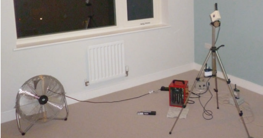
Fig. 11.5 An example of a typical coheating setup: electrical resistance heater with thermostatic control to maintain constant internal temperature, electricity and temperature logging equipment and a circulation fan to ensure air temperature uniformity in the zone
