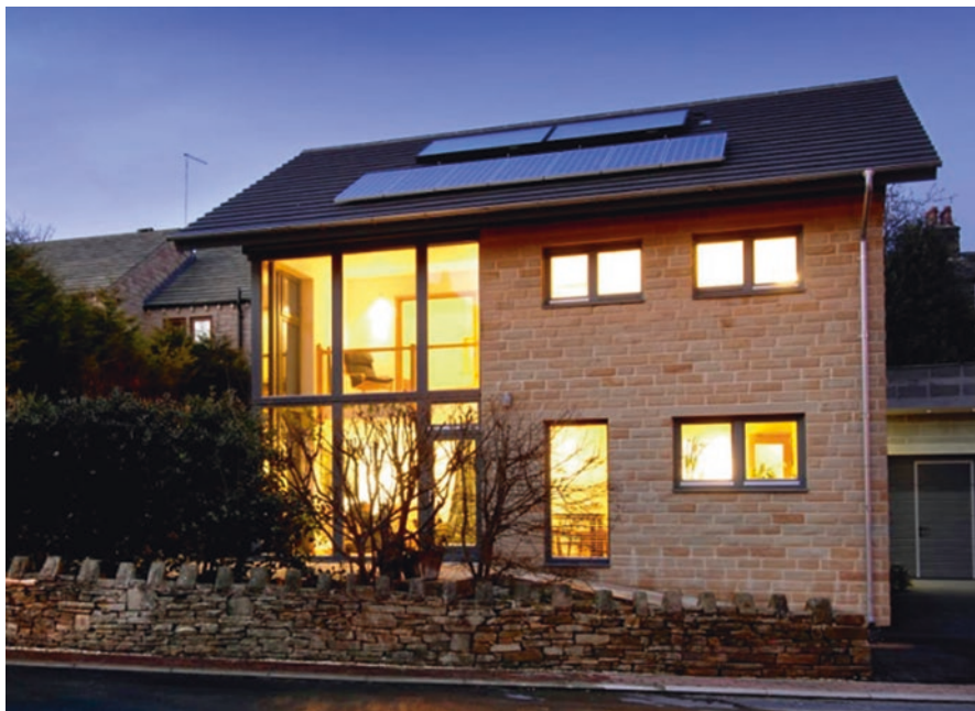
Fig. 11.8 Denby Dale Passivhaus (Green Building Store 2017)
