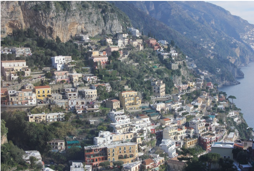
Fig. 3.6 Positano, on the Amalfi coast in Italy, is built on a sloping mountain respecting topography and benefiting from southern exposure
