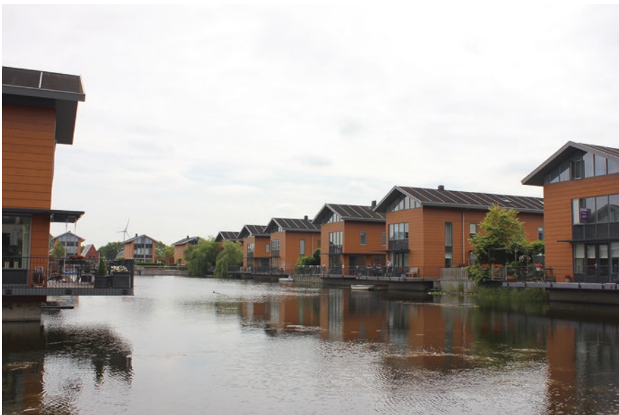
Fig. 3.22 Gabions are used to prop up canal facing buildings in the Netherlands
