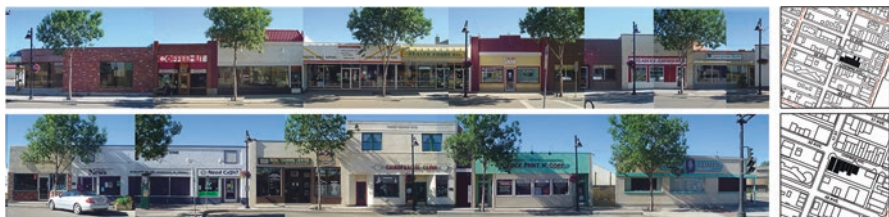
Fig. 3.27 Street façades on Chipman Avenue in Ponoka
