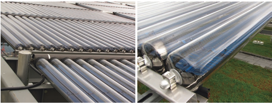
Fig. 5.17 The evacuated-tube collector system is an efficient technology which uses a series of parallel glass tubes filled with small amounts of antifreeze sealed in a small central copper pipe
