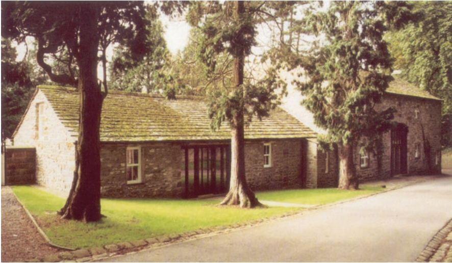
Fig. 7.6 The Pinetum Pavilion in the Broughton Hall Estate, Skipton, UK, from which companies work long distance taking advantage of digital communication
