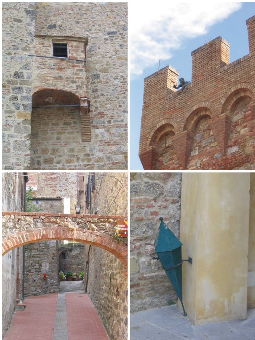
Fig. 6.11 Heritage buildings need to be restored with great care to avoid weathering and degradation of facades and to match the careful construction used at the time of their initial construction as was the case in the centre of Casole d'Elsa, Italy
