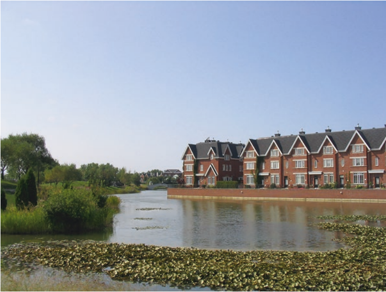
Fig. 4.19 A town could also introduce retaining ponds and wetlands to store the accumulated rainwater which may be used for recreation
