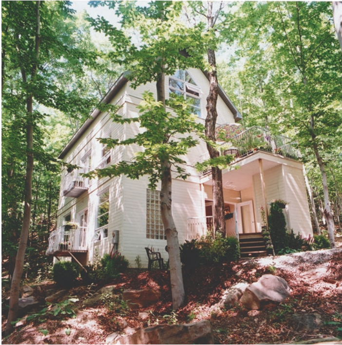
Fig. 3.9 In a rocky terrain, homes can be constructed on-grade avoiding excavation
