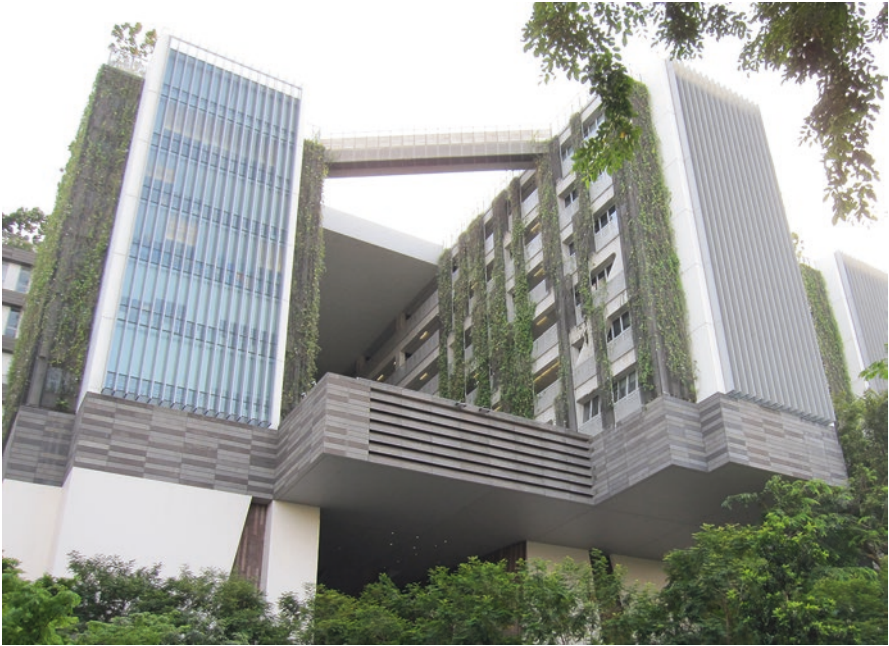
Fig. 3.16 Buildings with exterior green walls, also referred to as living walls , like this one in Singapore, may serve an important role in mitigating heat stress in urban areas
