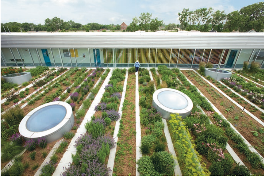
Fig. 3.18 Unused rooftops can accommodate significant potential to contribute to the food supply in small towns particularly in isolated northern communities, where food has to travel vast distances
