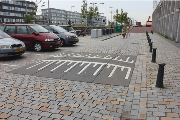
Fig. 4.16 Speed bumps and special paving materials in parking areas will alert drivers and lower speed
