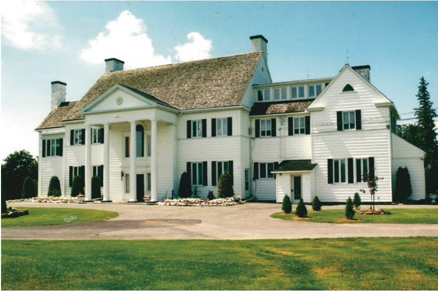
Fig. 3.3 A large estate that was built in the early 1900s as a summer residence in Senneville, a waterfront community near Montreal
