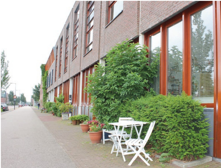
Fig. 5.6 Window placement, unit alignment, and landscaping can aid in reducing the perception of crowdedness
