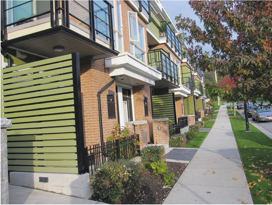
Fig. 6.12 By creating attractive and affordable housing close to amenities, an area can be renewed to offer a multitude of opportunities both for the residents and the surrounding community as was the case in North Vancouver, British Columbia, Canada
