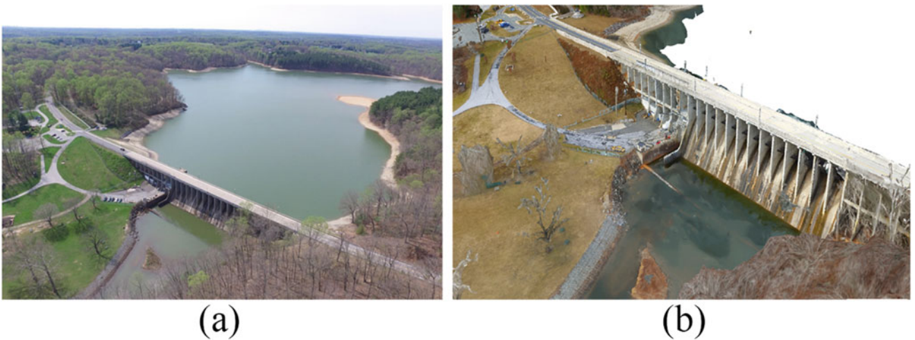
Fig. 26.1 (a) The Brighton Dam; (b) Dense 3D point cloud (January'17 dataset)
