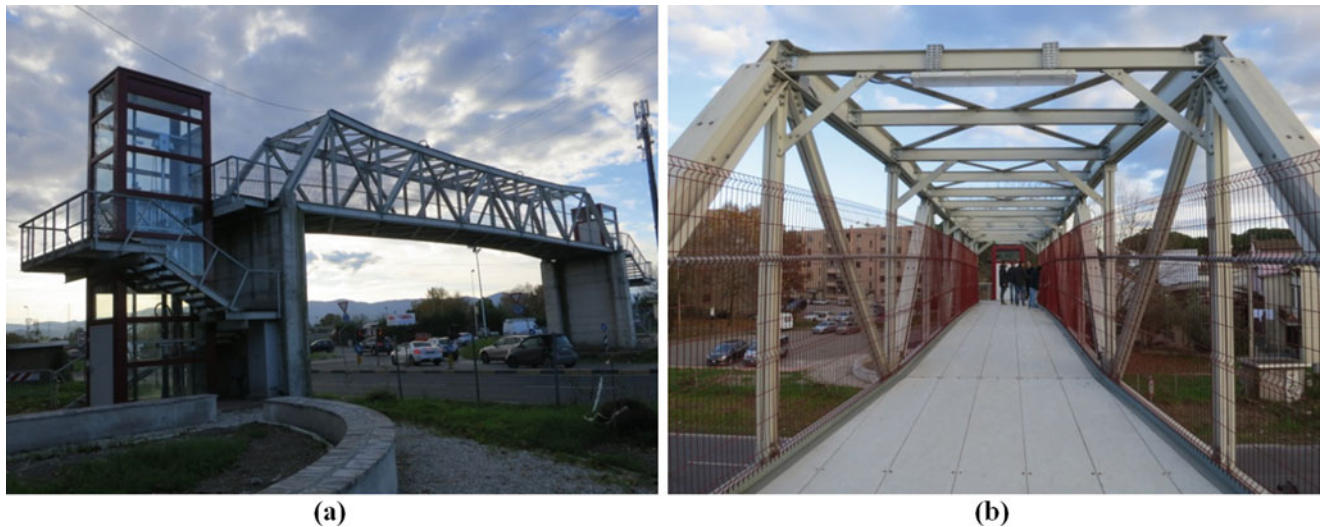
Fig. 22.1 The Prato Bridge: (a) side view; (b) deck view
