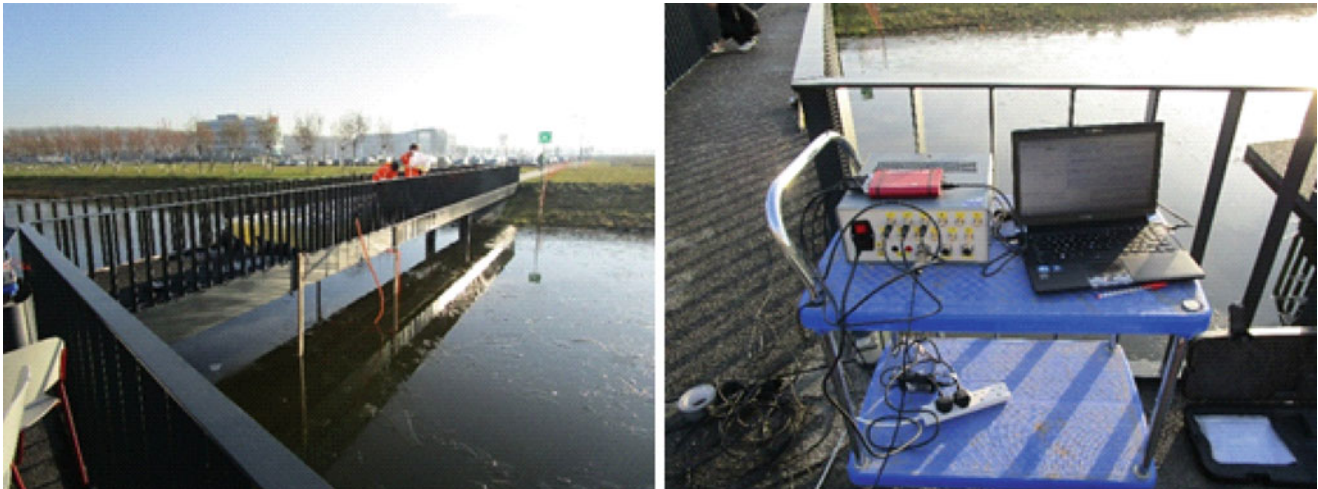
Fig. 19.1 Bridge 1 – left: side view and right: data acquisition station
