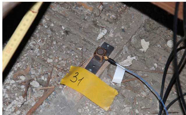
Fig. 14.16 MP 31 on top of the (central) lathing between cross girders 10 and 20. The state of health of the plastered reed layer being nailed to the lathing can also be seen
