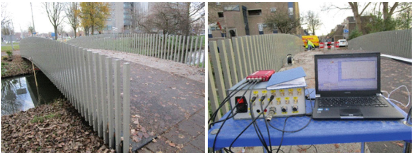
Fig. 19.2 Bridge 2 – left: side view and right: data acquisition station
