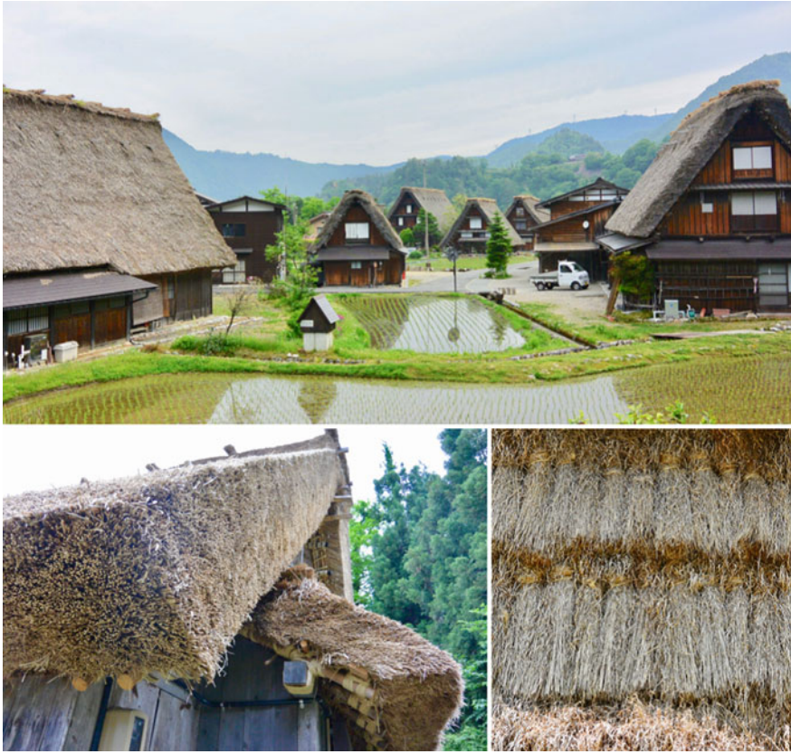
Fig. 3 Roof covered by grasses. The area, Shirakawa-go in Gifu Prefecture, has been designated as world cultural heritage (June 3, 2014)
