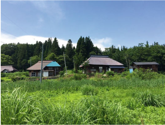
Fig. 1 Traditional folk houses in Karayama village (2 July 2015), one of the villages studied in Iiyama City in central Japan. Their original thatched roofs have been covered with tin allow the accumulated snow to slide down naturally
