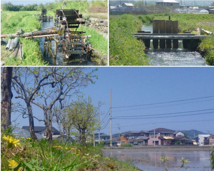
Fig. 5 Traditional irrigation system for rice cropping at Komatsushima in Tokushima Prefecture (April 17, 2012)
