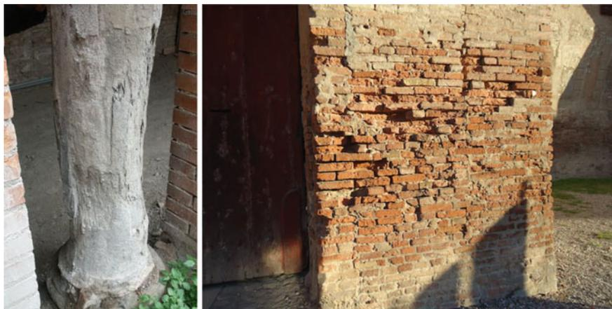
**Fig. 1.3** Examples of damages due to rising damp in a sandstone column (left) and a brick masonry (right). The deterioration patterns are due to a combination of salt crystallisation cycles and frost damage, both to be ascribed to the presence of moisture in the materials pores (*Photos Elisa Franzoni*)
