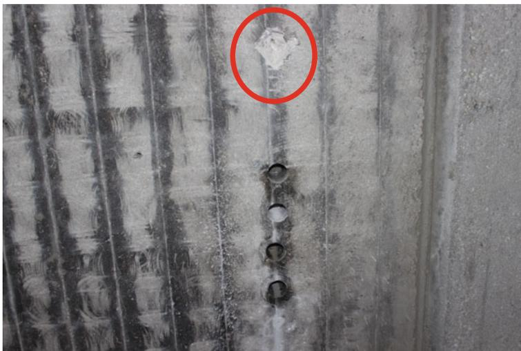
**Fig. 19.18** Sampling points for moisture balance measurements
