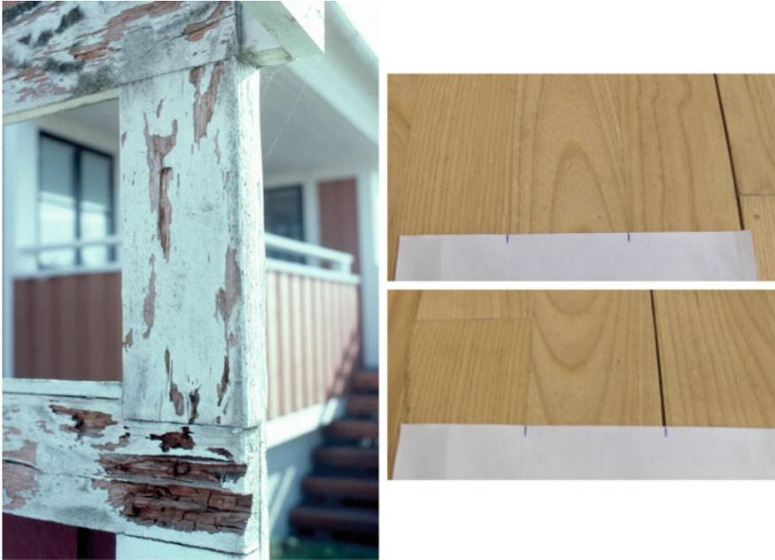
**Fig. 1.4** Examples of damages in wood structures due to too high moisture contents. Root decay in an outdoor timber structure with a non-suitable paint system (left) (*Photo Stefan Hjort*) and large gaps between floor tiles (right) (*Photo Lars-Olof Nilsson*). The board in the bottom centre has been compressed by swelling too much. The two marks show the width of the other tiles that were not compressed but shrank reversible after swelling
