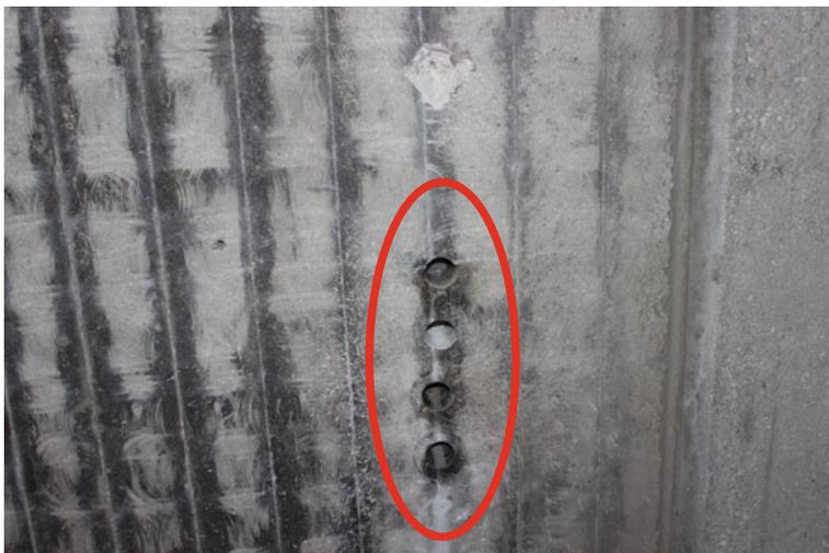
**Fig. 19.16** Coring area for gravimetric measurements
