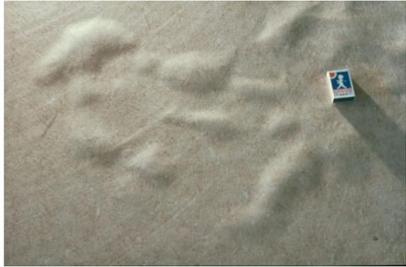
**Fig. 1.2** An example of a deteriorated concrete structure due to internal expansion from alkali-aggregate reactions that require a certain moisture level for the alkalis to reach the reactive aggregate. The structure is covered to protect against rain (*Photo Lars-Olof Nilsson*)
