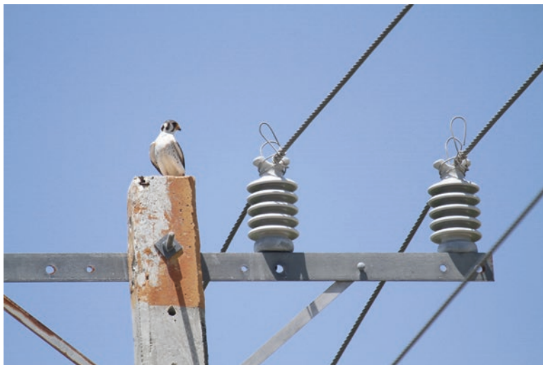
Fig. 12.5 Small raptors such as American kestrels can be at risk on poles with metal-grounded crossarms
