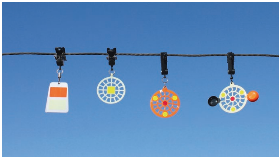
Fig. 12.14 Active wire markers: FireFly (left), BirdMark (middle left), CROCFast Static (middle right) and CROCFast Dynamic Diverter (right)
