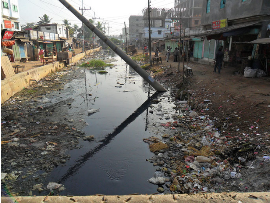
Fig. 12 Water pollution in the city areas due to careless throwing of wastages in the drainage systems
