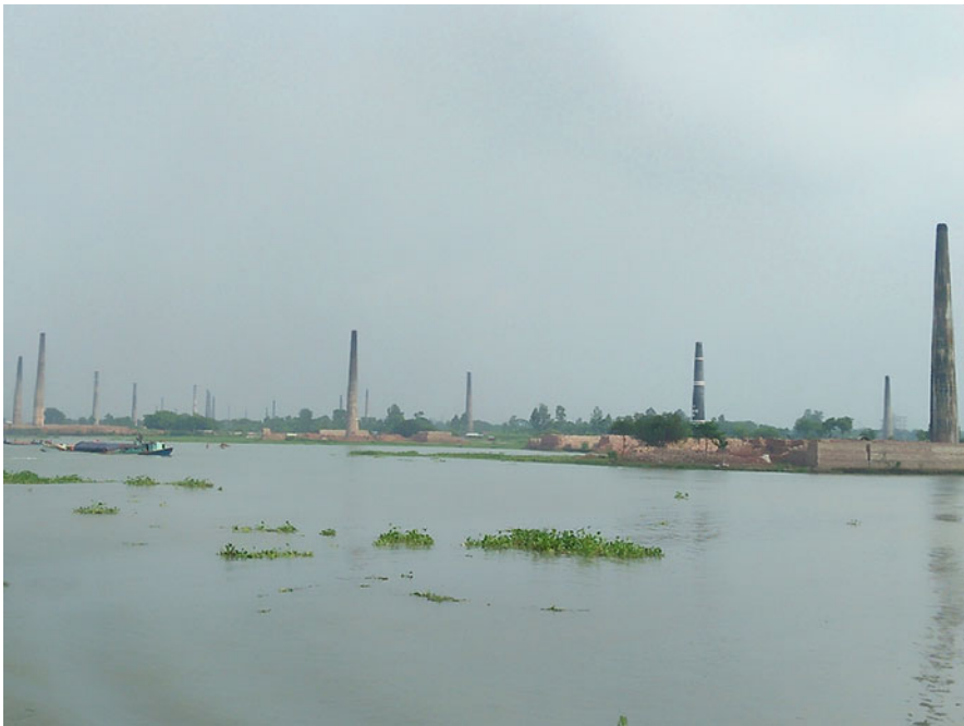
Fig. 3 Unplanned brick field construction on the bank of Buriganga River
