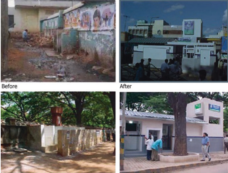
Plate 6.2 Location before and after the construction of Nirmala Toilets
