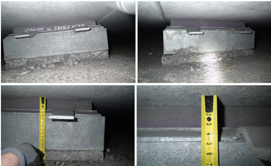
Fig. 2. Visual inspection of discrete bearings
