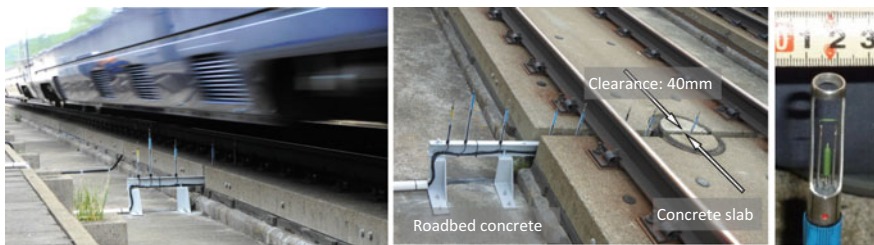
Fig. 1 Example of rolling stock passing over hot-wire anemometers installed on slab track
