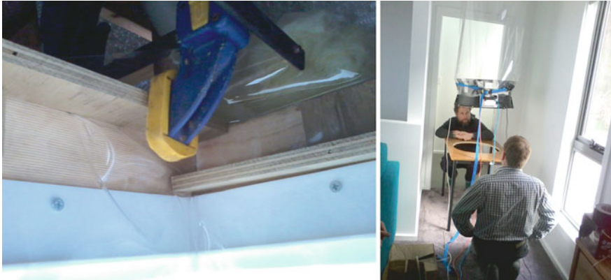
Fig. 11 Blower door apparatus modified for testing roof cavity
