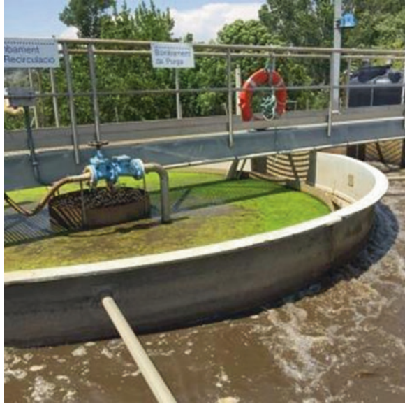
Fig. 3.15 Activated sludge wastewater treatment plant
