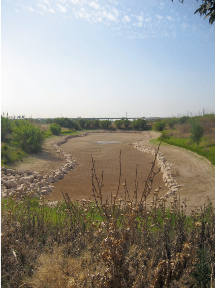
Fig. 3.8 Sedimentation pond
