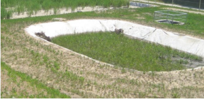
Fig. 3.30 Sludge reed bed
