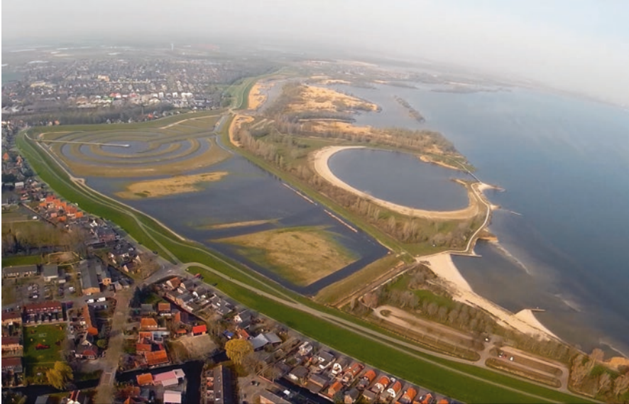
Fig. 3.2 Aerial view of Lake Ijsselmeer showing inland shore (Source: Deltares)
