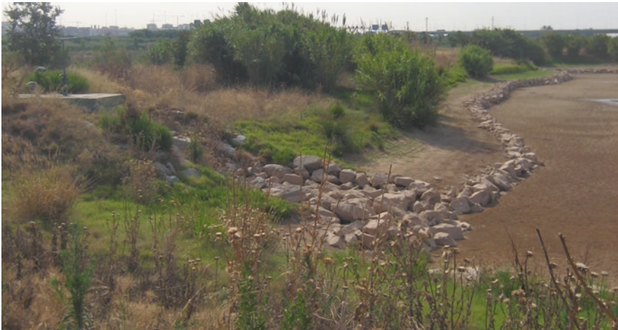
Fig. 3.5 Inlet from Llobregat river
