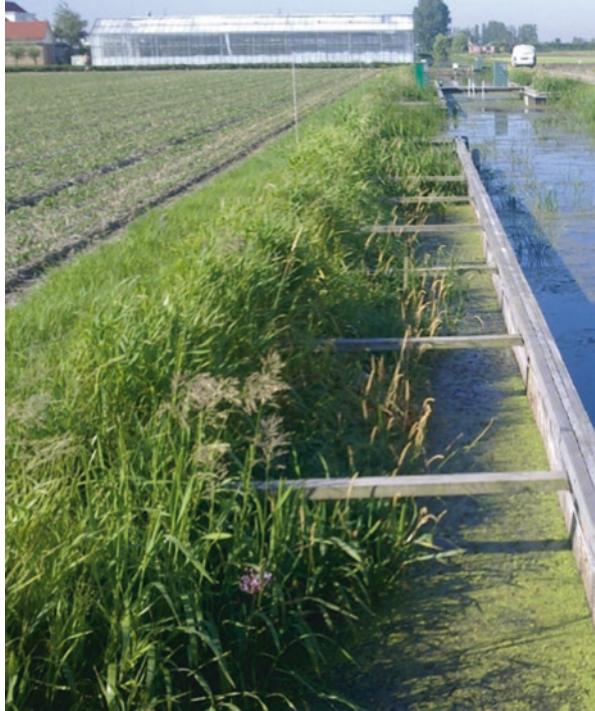
Fig. 3.25 Purifying bench for phosphate removal
