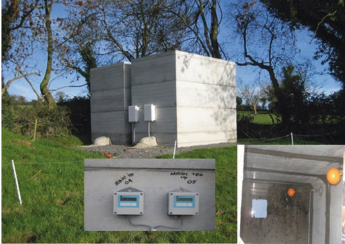
Fig. 3.43 Rainwater storage system with mains water back-up
