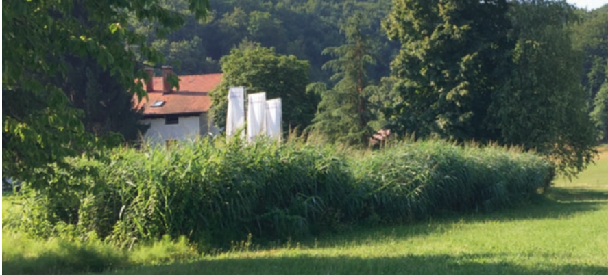
Fig. 3.33 Natural wastewater treatment system, fish processing factory, Slovenia
