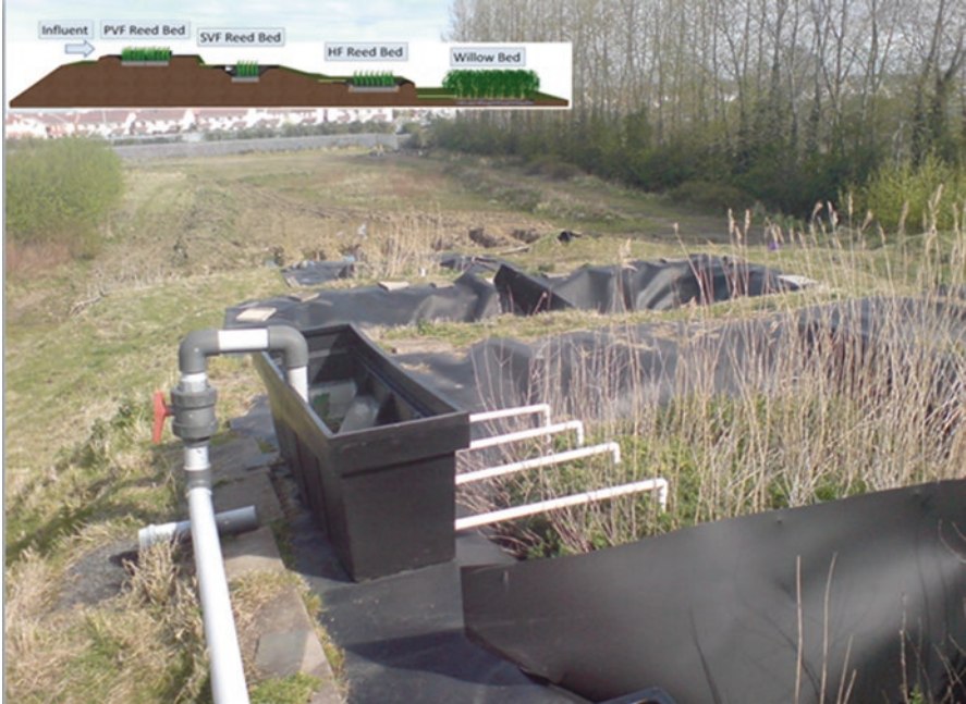
Fig. 3.46 Overview of treatment system showing PVF reed bed, SVF reed bed, HF reed bed and Willow bed
