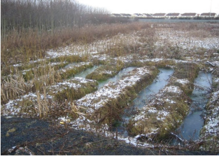
Fig. 3.48 System operating in winter 2012
