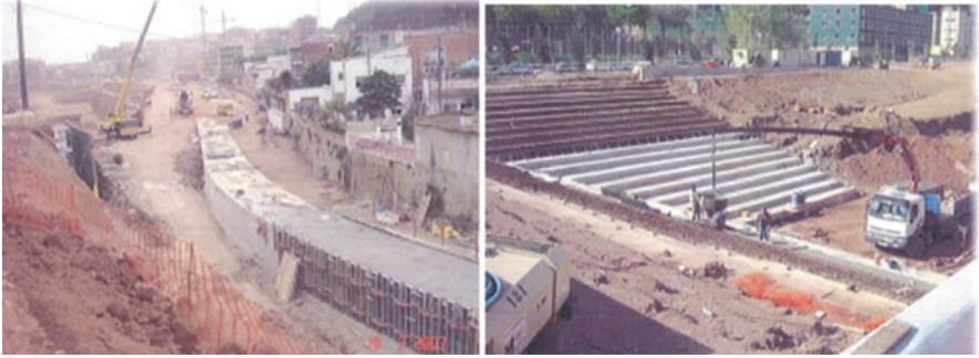
Fig. 3.20 Collector bypass
