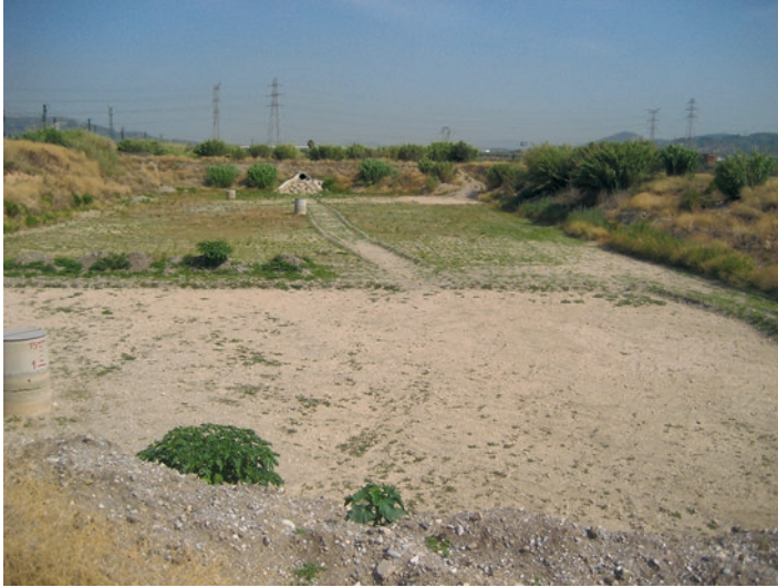
Fig. 3.6 Inlet from sedimentation pond and piezometer well
