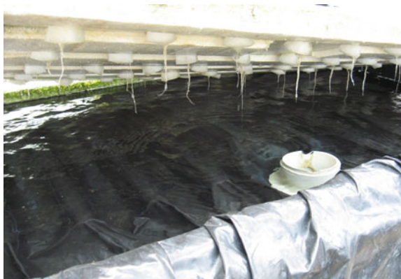
Fig. 7.18 The shallow water level in DRFT
