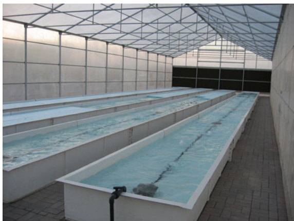
Fig. 7.6 Plant tanks in an aquaponic system where plants grow with bare roots
