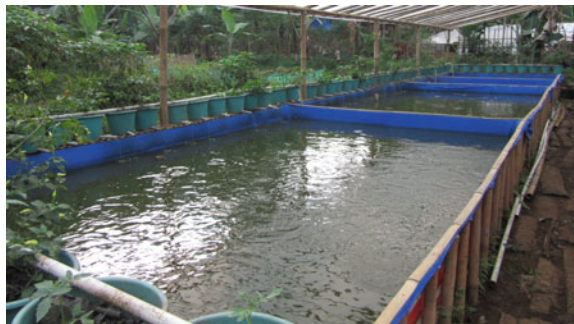
Fig. 7.9 Fish tanks made of liners and bamboo stakes
