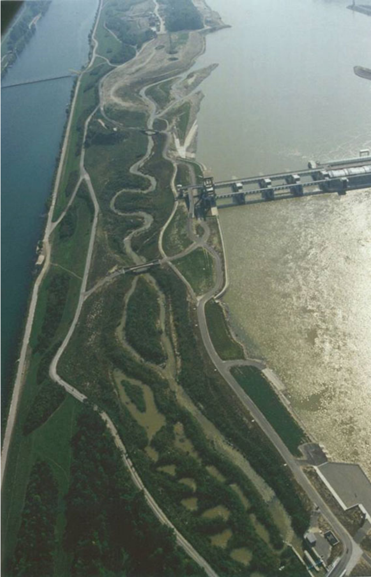
Fig. 24.7 Bypass channel system for fish migration at the power station “Freudenau” (Section 4) (courtesy of Verbund AG)
