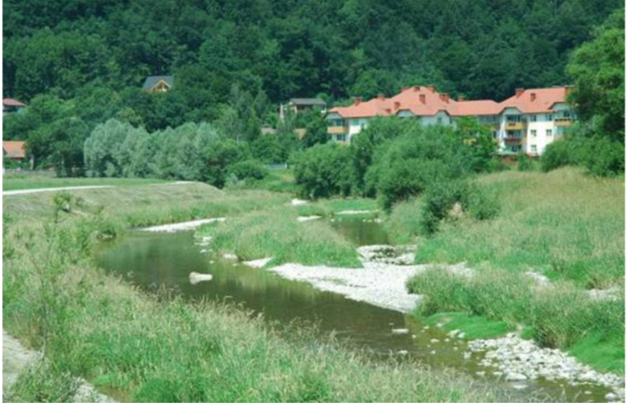
Fig. 4.7 Encroachment of vegetation into river channel, example residual flow stretch River Gölsen
