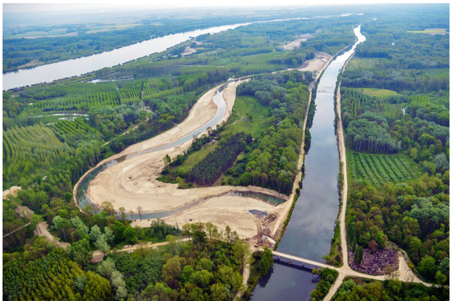
Fig. 15.4 Bifurcation of the newly excavated riverbed with the adjoining lowered floodplain terrain (left) from the old straight Traisen canal (right) prior to its flooding (in the background: Danube River; source: M. Haslinger and Verbund AG 2014)
