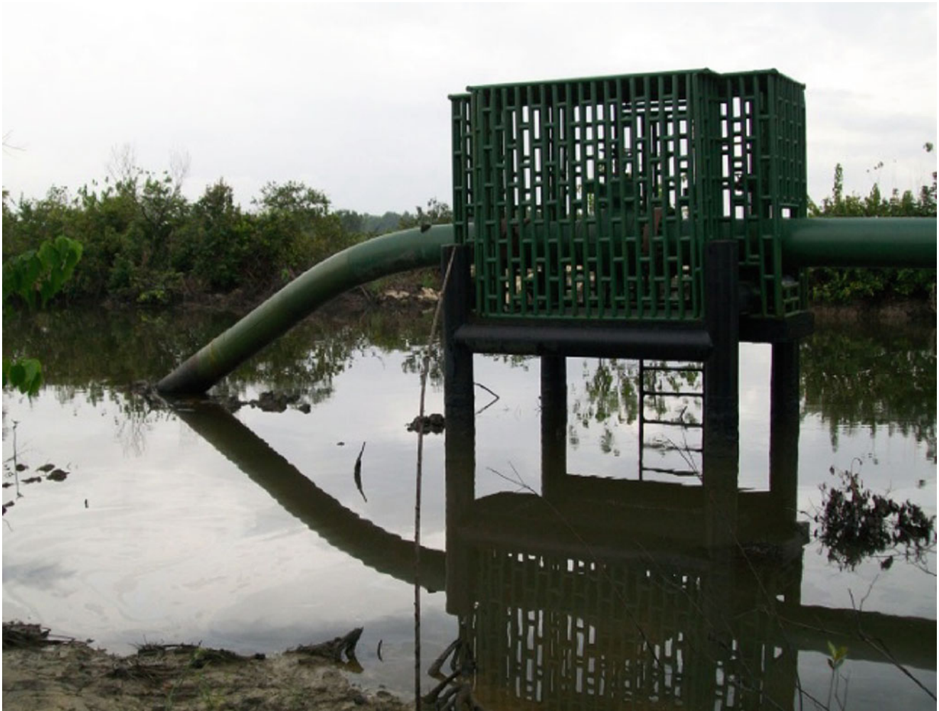
Fig. 12.6 Crude oil well-head located in a mangrove swamp in Buguma, Niger Delta Nigeria. It shows some sections of the mangrove forest already cleared to install rigs and pipes. Pipeline corrosion occurs several years after submergence under water (Credit: A.O. Numbere)
