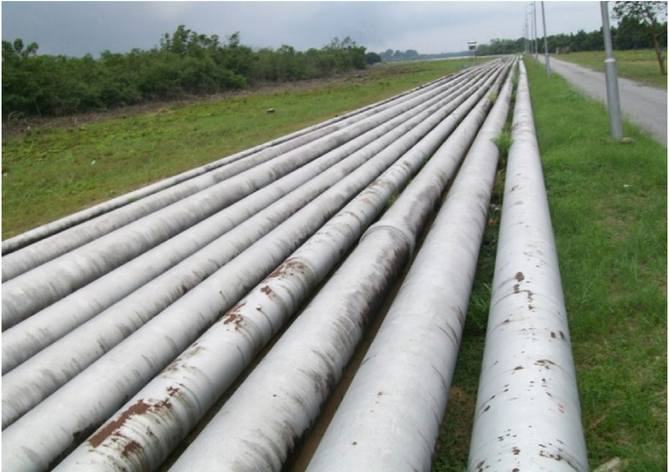
Fig. 12.5 Nickel/steel alloy pipelines (measuring between 8 and 10") starting from the refinery to the loading jetty at Okrika in the Niger Delta area of Nigeria. It has an approximate length of 16 km. Mangrove forest is found on the left and right sides while the middle area, which formerly had mangrove trees is now made bare to create a right of
