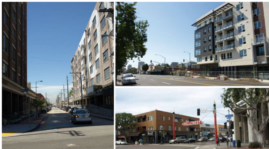
Fig. 4.9 URFSURB variants: (left) loft conversion of former industrial buildings, Skid Row, Los Angeles; (upper right) new apartment block, East Village, San Diego—both locations are linked structurally and functionally to the respective urban center. In contrast, Hillcrest (lower right), some 5 km north of downtown San Diego, reveals a typically urban pattern of public and private service provision (Photos Olaf Kühne)
