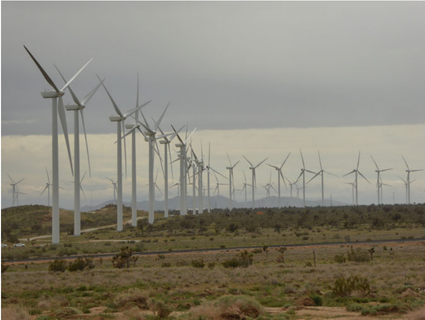
Fig. 5.15 Wind farm on the borders of California’s Mojave Desert. In contrast with the decentralized European model, several hundred wind turbines—along with their side-effects on the landscape—are packed here into a relatively small space (Photo Olaf Kühne)
