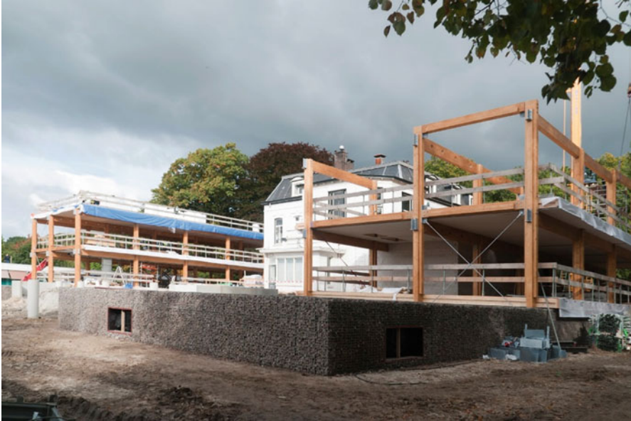
Fig. 12.3 Brummen Town Hall during construction (Photo Credit: Royal BAM Group nv)
