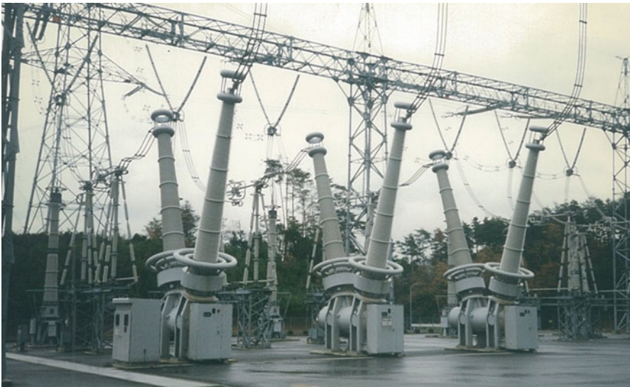
Fig. 2.33 550 kV 63 kA single-break SF 6 gas circuit breaker. (Courtesy of Chugoku Electric Power)
