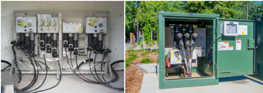
Fig. 2.43 27 kV, 630 A solid dielectric insulated switchgears: dry vault (left) and pad-mounted (right) applications. (Courtesy of G&W Electric Company)
