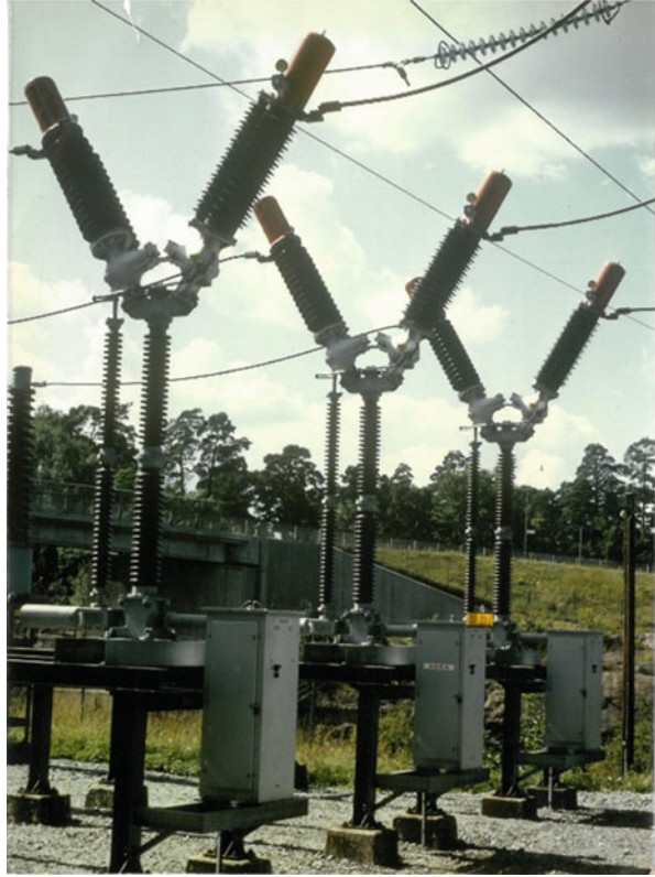
Fig. 2.27 245 kV 50 kA live tank oil circuit breaker. (Courtesy of ABB, product of ASEA in 1985)
