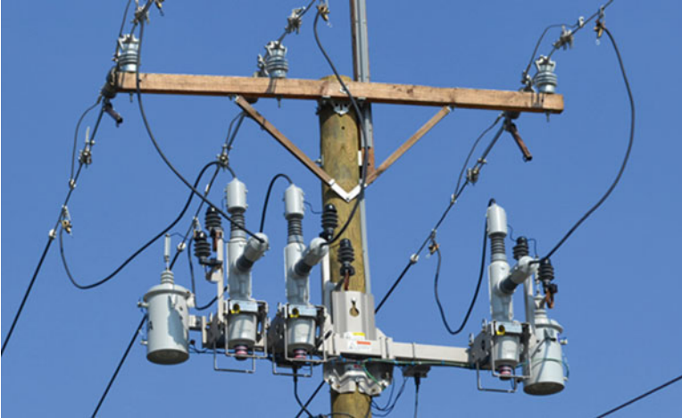
Fig. 2.41 Pole top recloser with solid dielectric insulation in accordance with IEEE C37.60/IEC 62271–111. (Courtesy of G&W Electric Company)
