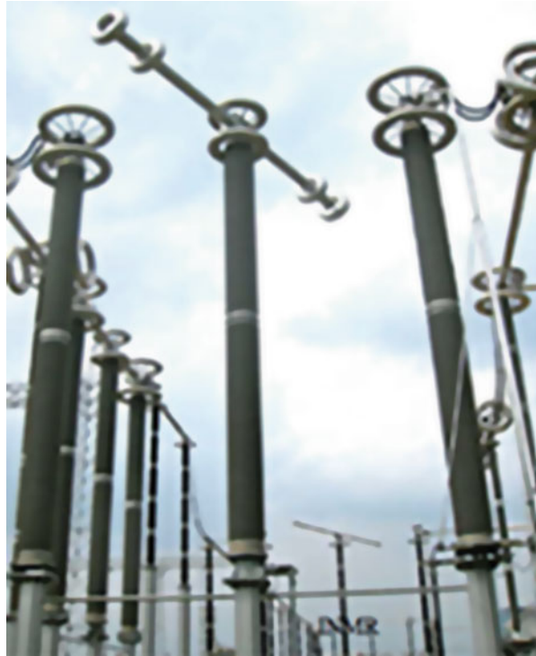
Fig. 16.36 800 kV DC DS corresponding to group C (Mikli et al. 2012). (Courtesy of Siemens)
