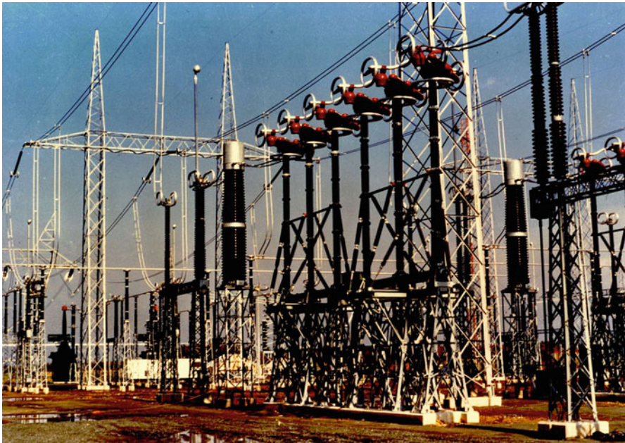
Fig. 5.21 Latest generation 800 kV air blast circuit breaker. (Courtesy of GE Grid Solutions, produced by Alstom)
