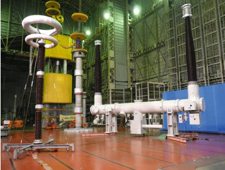
Fig. 10.2 Dielectric withstand performance tests with 550 kV H-GIS
