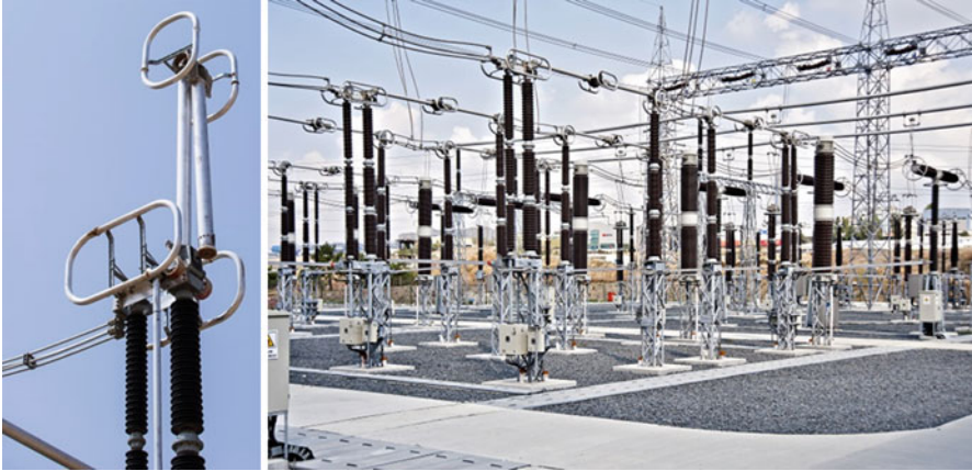
Fig. 9.16 Knee-type disconnecting switch. (Courtesy of GE Grid Solutions)
