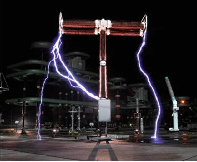
Fig. 10.12 Lightning impulse voltage test with 420 kV live tank circuit breaker. (Courtesy of Siemens)
