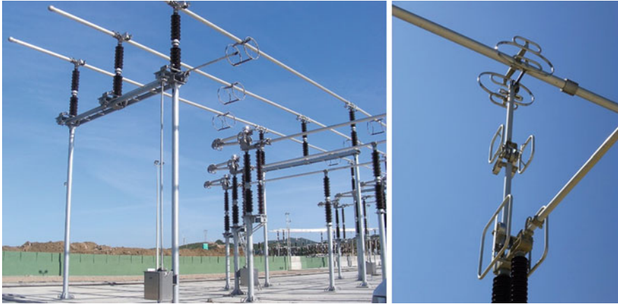
Fig. 9.18 Semi-pantograph disconnecting switch. (Courtesy of Coelme-Egic)
