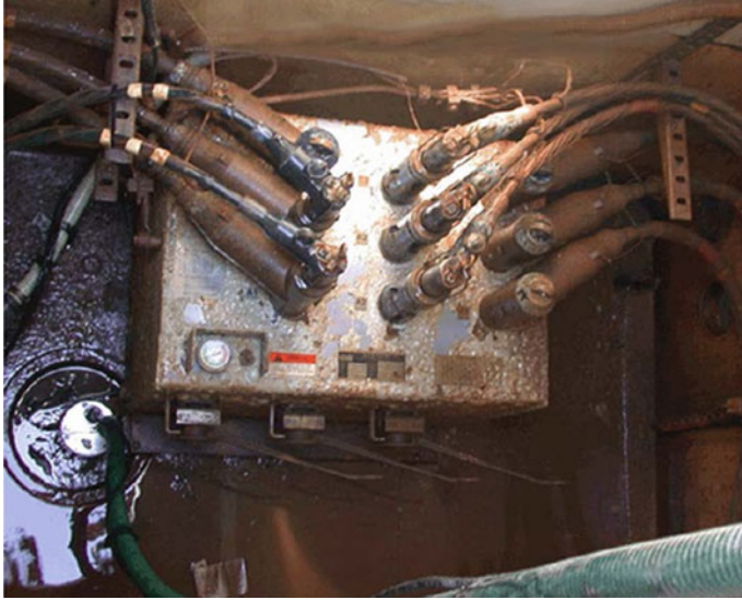
Fig. 2.42 27 kV 630 A SF 6 insulated dead tank switch. (Courtesy of G&W Electric Company)
