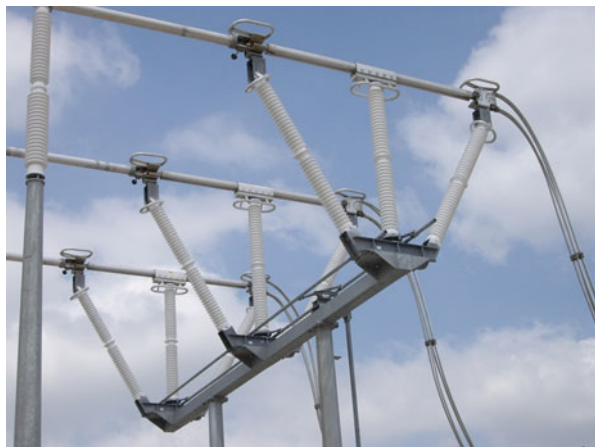
Fig. 9.15 Double side break disconnecting switch. (Courtesy of GE Grid Solutions)
