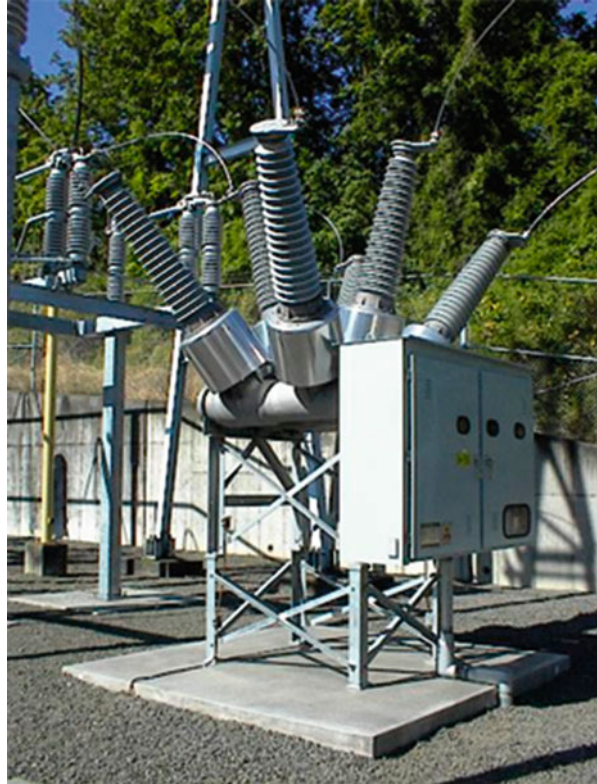
Fig. 6.23 145 kV dead tank gas circuit breaker. (Courtesy of Portland G&E)
