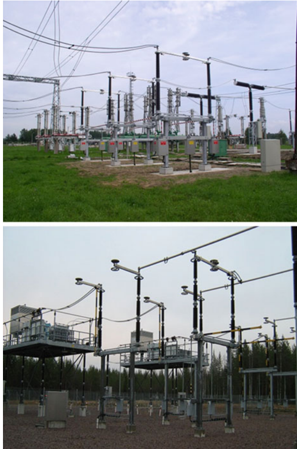
Fig. 9.14 Center side break disconnecting switch. (Courtesy of Hapam B.V.)
