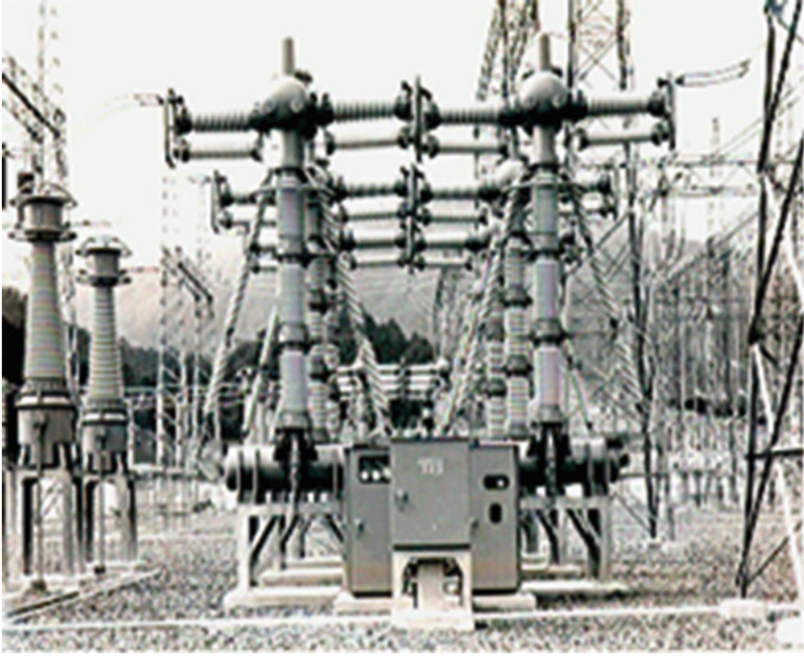
Fig. 6.20 300 kV double-pressure-type live tank gas circuit breaker (1966)
