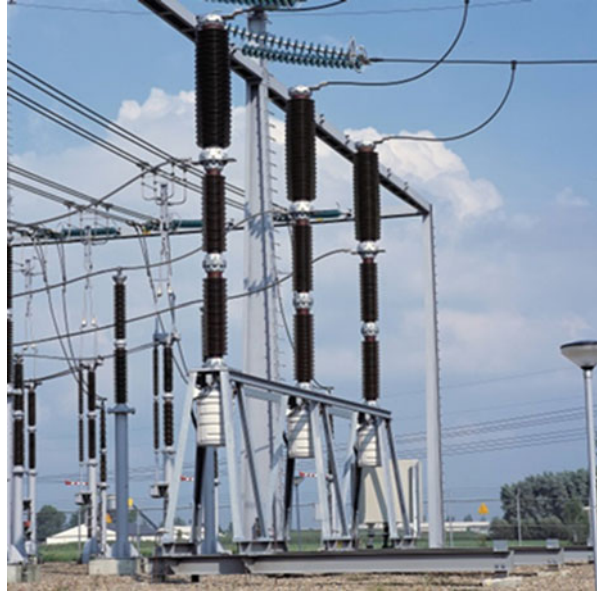
Fig. 2.10 Three single-phase independent operated gas circuit breakers. (Courtesy of TenneT TSO B.V)
