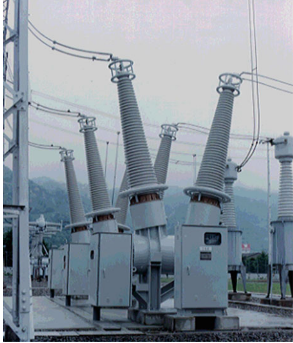
Fig. 6.22 300 kV single break dead tank gas circuit breaker (1981). (Courtesy of Kansai Electric Power)
