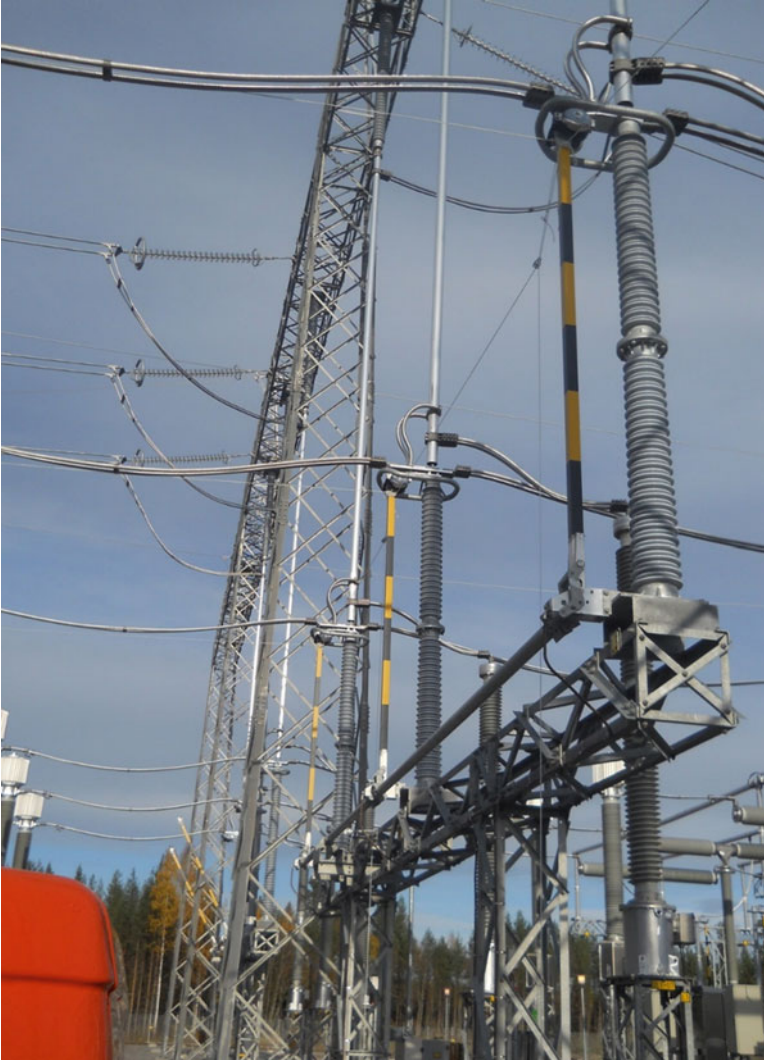
Fig. 9.22 Earthing switch. (Courtesy of Hapam B.V.)
