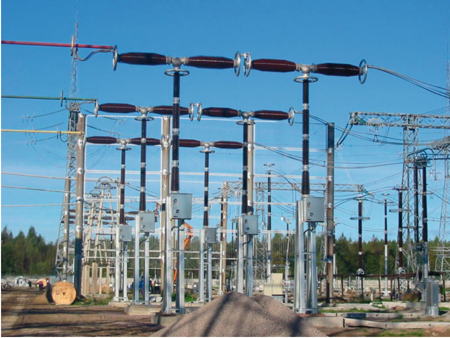
Fig. 6.21 420 kV single pressure-type live tank gas circuit breaker. (Courtesy of GE Grid Solutions)
